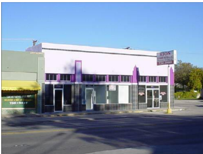
Façade improvements can go a long way towards increasing value.
