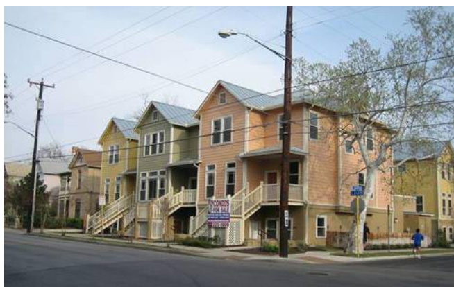
Residential buildings 2-3 stories high will add diversity to the urban village.
