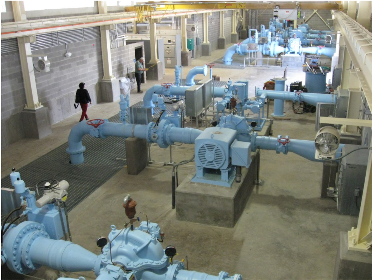
Sendera Ranch Pump Station
