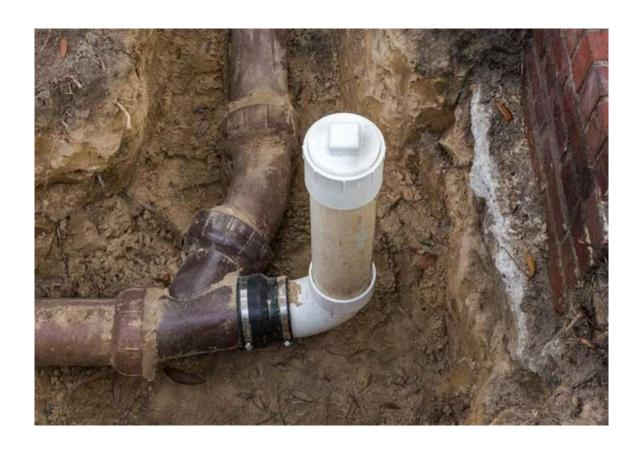
Sanitary sewer service will not be interrupted. New sewer cleanouts will be installed at the property line.
