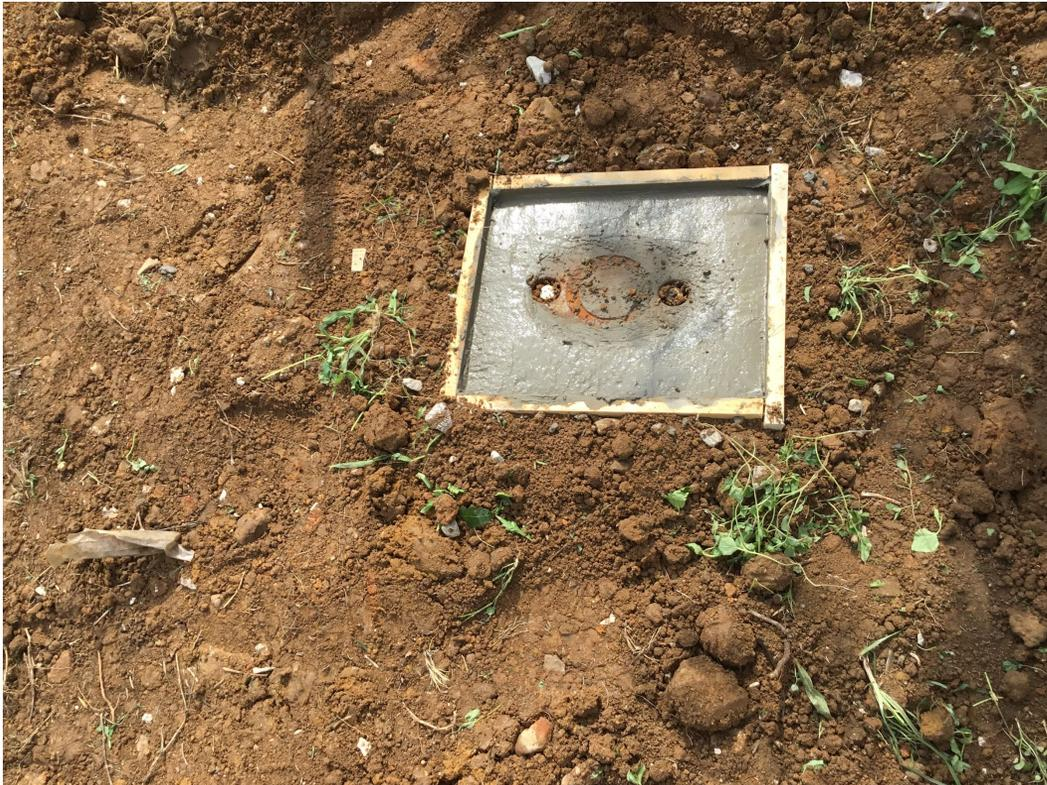
The sewer cleanout provides crews easy access if a backup or blockage occurs.
