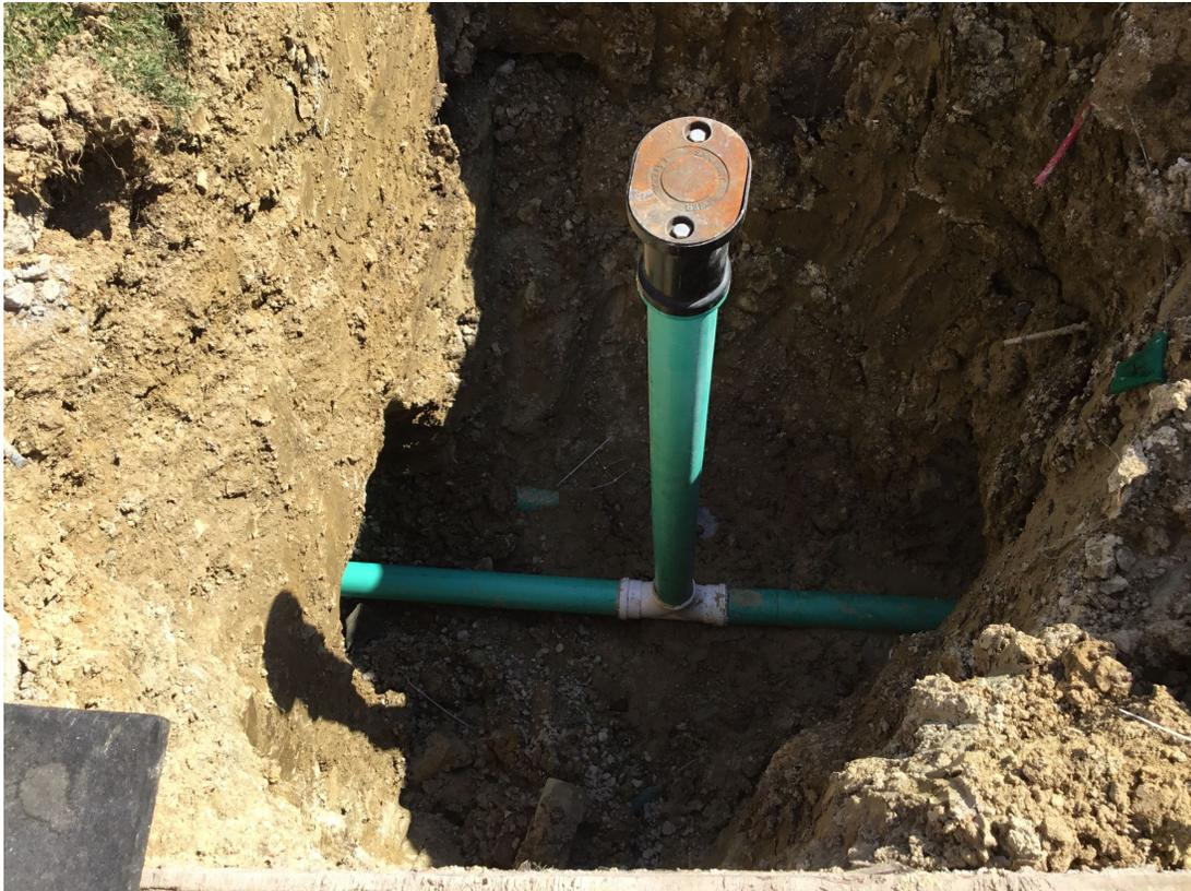
The City side of the line starts at the main in the street and goes to the customer's sewer cleanout.
