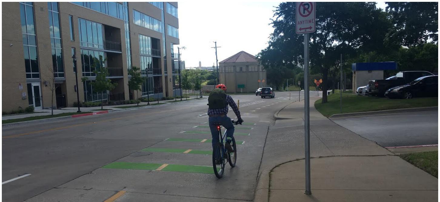
Figure 5. A bicyclist rides in a two-way bike lane with green paint marking the driveway conflict. Photo Credit: City of Fort Worth
