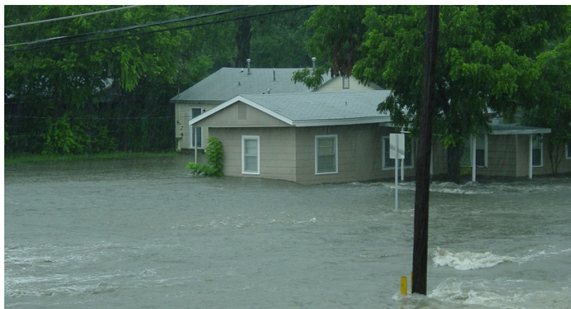
Figure 4: Flooding in Seminary Hills – 2004
