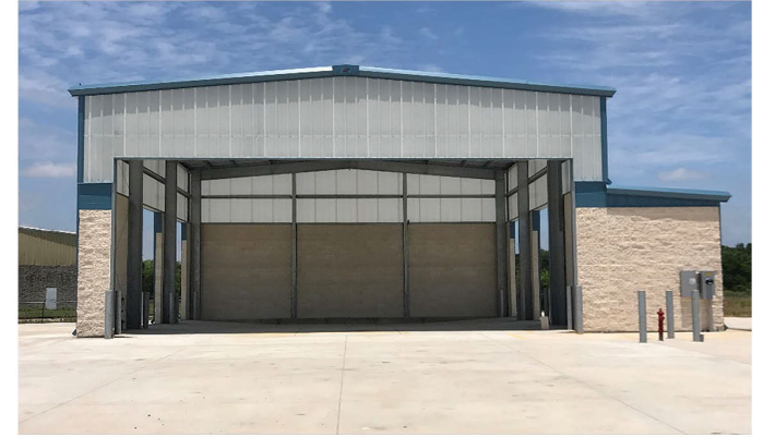
Support street sweeper operations with new wash bay facilities.
