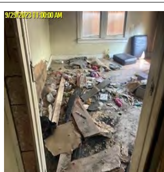
Comp/Insp Date: 9/29/2023 Bedroom
