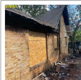
Line Item Date: 9/29/2023 Completion After Photo Photos
