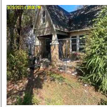
9/29/2023 1:09:00 PM Comp/Insp Date: 9/29/2023 Bid Photo REMOVE EXTERIOR DEBRIS PER CU YD
