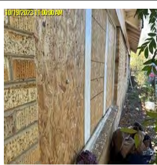
Comp/Insp Date: 10/19/2023 Front Right View
