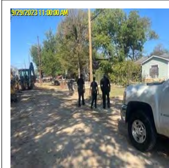
Comp/Insp Date: 9/29/2023 Front View
