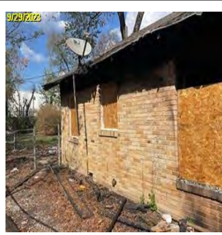
9/29/2023 Line Item Date: 9/29/2023 Completion After Photo Photos
