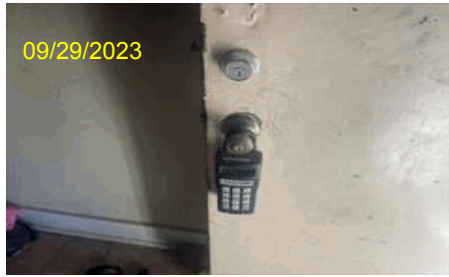
Image Type:Completion Before Photo Address:4433 Virginia Ln City,State Zip:Forth Worth, TX 76103 Line Item Desc:Lock Box
