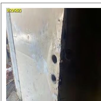
Line Item Date: 9/29/2023 Completion During Photo Lock Change
