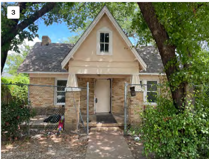
Project: 4433 Virginia Ln, Fort Worth, TX 76103 Date: 7/13/2023, 1:27pm Creator: Enrique
