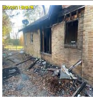
Comp/Insp Date: 9/29/2023 Bid Photo Structural Inspection
