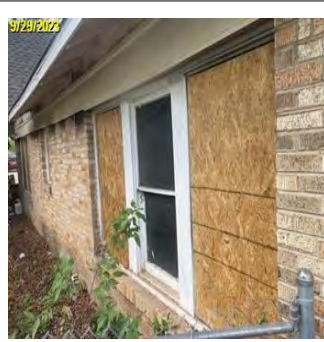
9/29/2023 Line Item Date: 9/29/2023 Completion After Photo Photos
