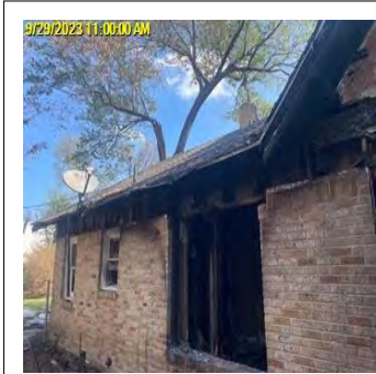
Comp/Insp Date: 9/29/2023 Front Right View
