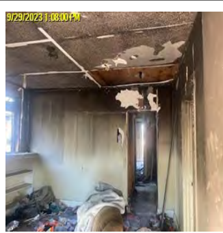
Comp/Insp Date: 9/29/2023 Bid Photo Structural Inspection
