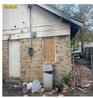
Line Item Date: 9/29/2023 Completion After Photo Photos
