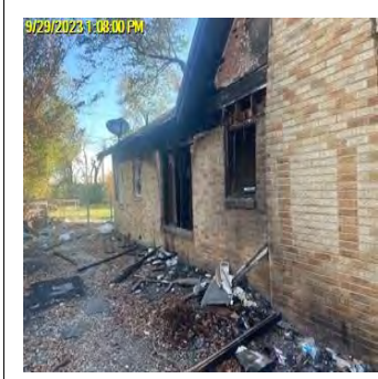
9/29/2023 1:08:00 PM Comp/Insp Date: 9/29/2023 Bid Photo REMOVE EXTERIOR DEBRIS PER CU YD
