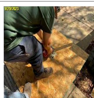
9/29/2023 Line Item Date: 9/29/2023 Completion During Photo Photos
