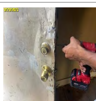
Line Item Date: 9/29/2023 Completion During Photo Lock Change
