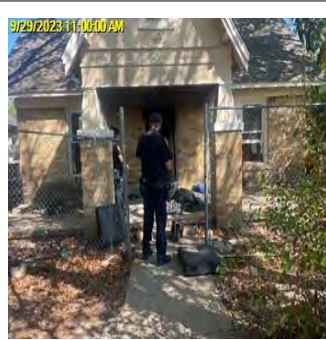
Comp/Insp Date: 9/29/2023 Front View
