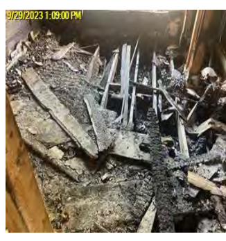
Comp/Insp Date: 9/29/2023 Bid Photo REMOVE INTERIOR DEBRIS PER CU YD
