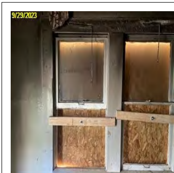
9/29/2023 Line Item Date: 9/29/2023 Completion After Photo Photos
