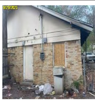
9/29/2023 Line Item Date: 9/29/2023 Completion After Photo Photos
