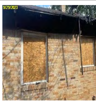
Line Item Date: 9/29/2023 Completion After Photo Photos
