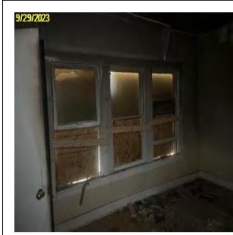
9/29/2023 Line Item Date: 9/29/2023 Completion After Photo Photos
