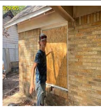
9/29/2023 Line Item Date: 9/29/2023 Completion During Photo Photos
