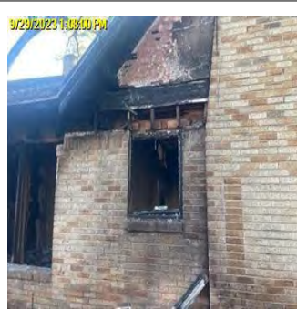
Comp/Insp Date: 9/29/2023 Bid Photo Structural Inspection
