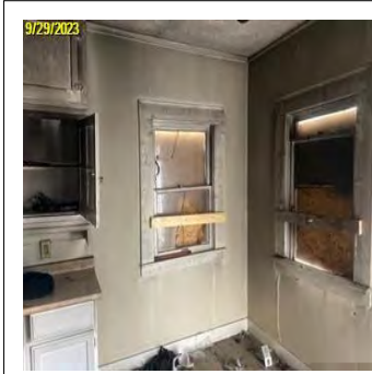
9/29/2023 Line Item Date: 9/29/2023 Completion After Photo Photos
