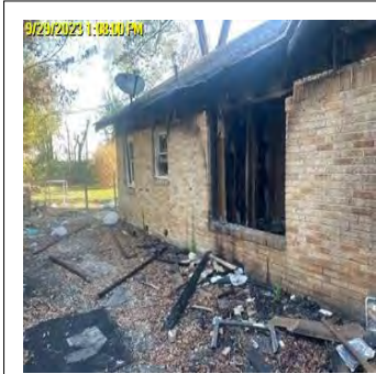
Comp/Insp Date: 9/29/2023 Bid Photo Structural Inspection
