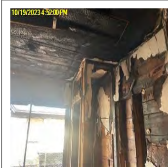
Comp/Insp Date: 10/19/2023 Bid Photo Structural Inspection
