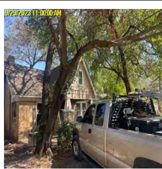
Comp/Insp Date: 9/29/2023 Front View
