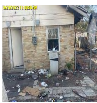
Comp/Insp Date: 9/29/2023 Exterior Doors
