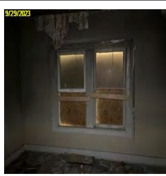
9/29/2023 Line Item Date: 9/29/2023 Completion After Photo Photos
