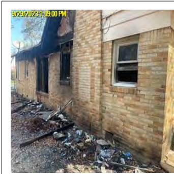
Comp/Insp Date: 9/29/2023 Bid Photo REMOVE EXTERIOR DEBRIS PER CU YD
