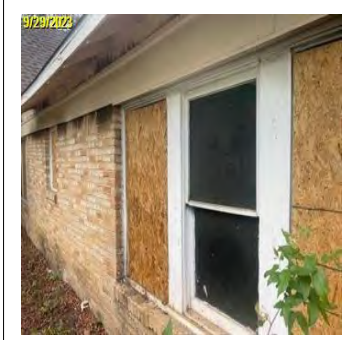
Line Item Date: 9/29/2023 Completion After Photo Photos
