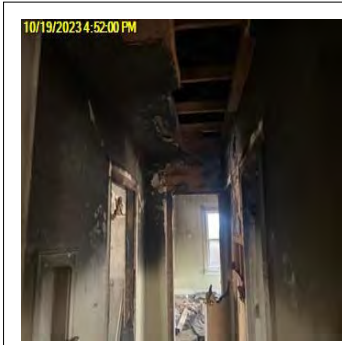
Comp/Insp Date: 10/19/2023 Bid Photo Structural Inspection
