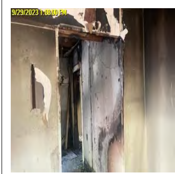
Comp/Insp Date: 9/29/2023 Bid Photo Structural Inspection
