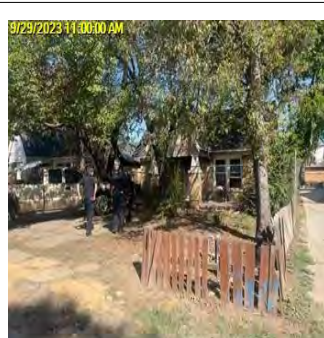
Comp/Insp Date: 9/29/2023 Front View
