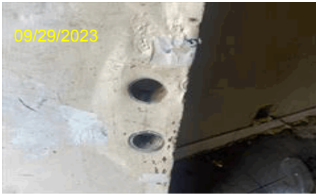
Image Type:Completion During Photo Address:4433 Virginia Ln City,State Zip:Forth Worth, TX 76103 Line Item Desc:Lock Change
