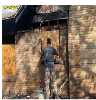
Line Item Date: 9/29/2023 Completion During Photo Photos
