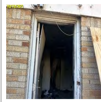
Line Item Date: 10/19/2023 Completion During Photo Board All Accessible Openings
