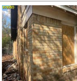
Line Item Date: 9/29/2023 Completion After Photo Photos
