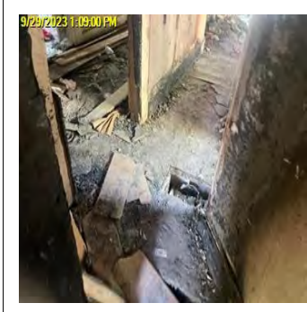
Comp/Insp Date: 9/29/2023 Bid Photo REMOVE INTERIOR DEBRIS PER CU YD
