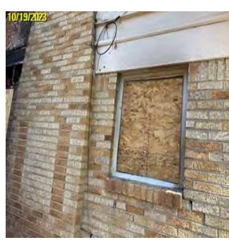
Line Item Date: 10/19/2023 Completion After Photo Board All Accessible Openings
