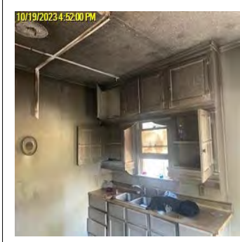
Comp/Insp Date: 10/19/2023 Bid Photo Structural Inspection
