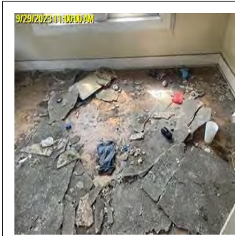
Comp/Insp Date: 9/29/2023 Bedroom
