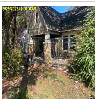
Comp/Insp Date: 9/29/2023 Front View
