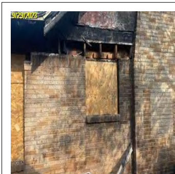
Line Item Date: 9/29/2023 Completion After Photo Photos
