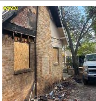
Line Item Date: 9/29/2023 Completion After Photo Photos
