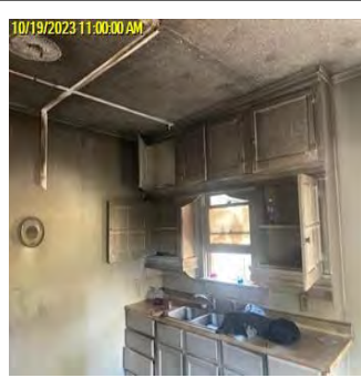
Comp/Insp Date: 10/19/2023 Kitchen
