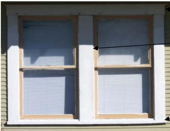
*Always double the width of trim between paired windows. Make sure to include a wood drip cap above the trim and a wood sill. Drip caps help to prevent water from seeping behind the window unit and prevent water damage to the wall.*
