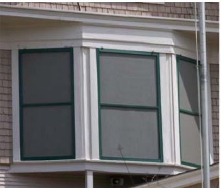
Solar screening is more opaque than traditional screening. This allows for more privacy while still allowing for air circulation. It will reduce the amount of light infiltration, by reflecting the sun's rays and because of its thickness it will help to trap heat in the winter months. The reflection of the sun ray's will also extend the life of your window unit.
