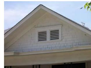
Gable vents are appropriate for structures that have gable roof forms. They come in a variety of shapes and sizes. They should be louvered and in a wood frame. Gable vents are inappropriate as a replacement for gables that feature decorative windows or stained glass.
