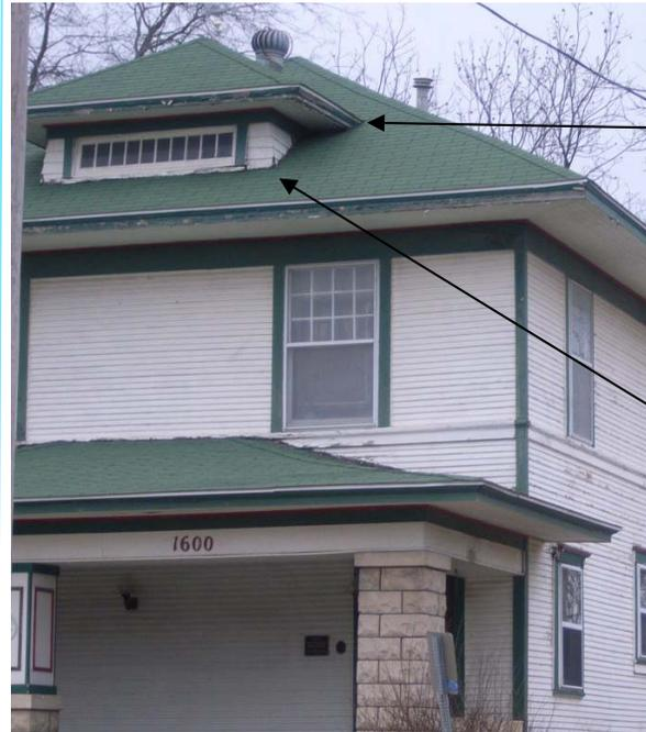
**Do** use modest proportions for both the roof and body. This dormer's eaves mimic the width of the main structure's eave but are proportional to the body of the dormer.
