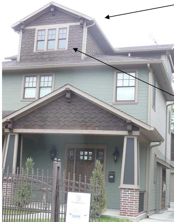
**Don't** replicate the main structure's eave line on the dormer or oversize the roof. It makes the dormer top heavy. The dormer roof proportion is typically 125% to 140% of the dormer body.
