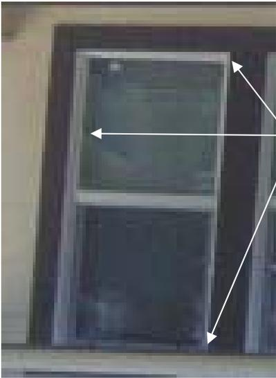
*If a wood window is deemed non-repairable give special attention when choosing a replacement. Consider material, size, grid pattern and installations. Material changes **MUST** be approved by the HCLC but are generally not approved. Replacement windows should be recessed mounted, meaning they are not flush with the exterior of the wall and fit the original opening. Often the dimensions are difficult to replicate, ask Staff for assistance.*
