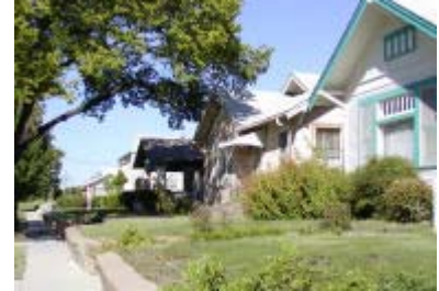
Near Southeast streetscape
