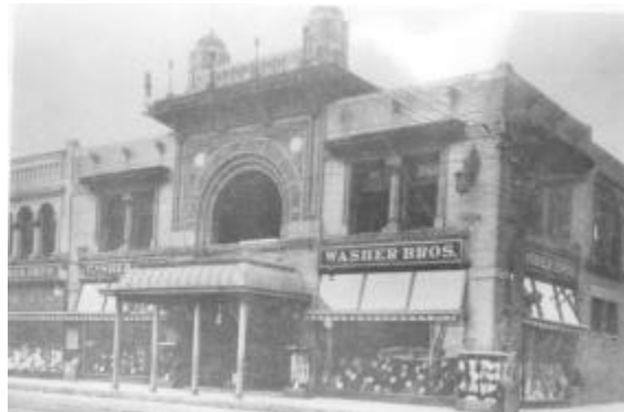
Façade rehabilitation programs help to preserve historic commercial buildings.
