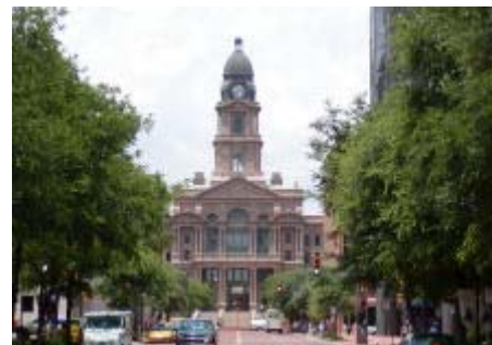
Tarrant County Courthouse
