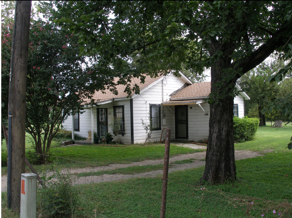
Resource Number 001, 1420 Carson Street, facing northeast.
