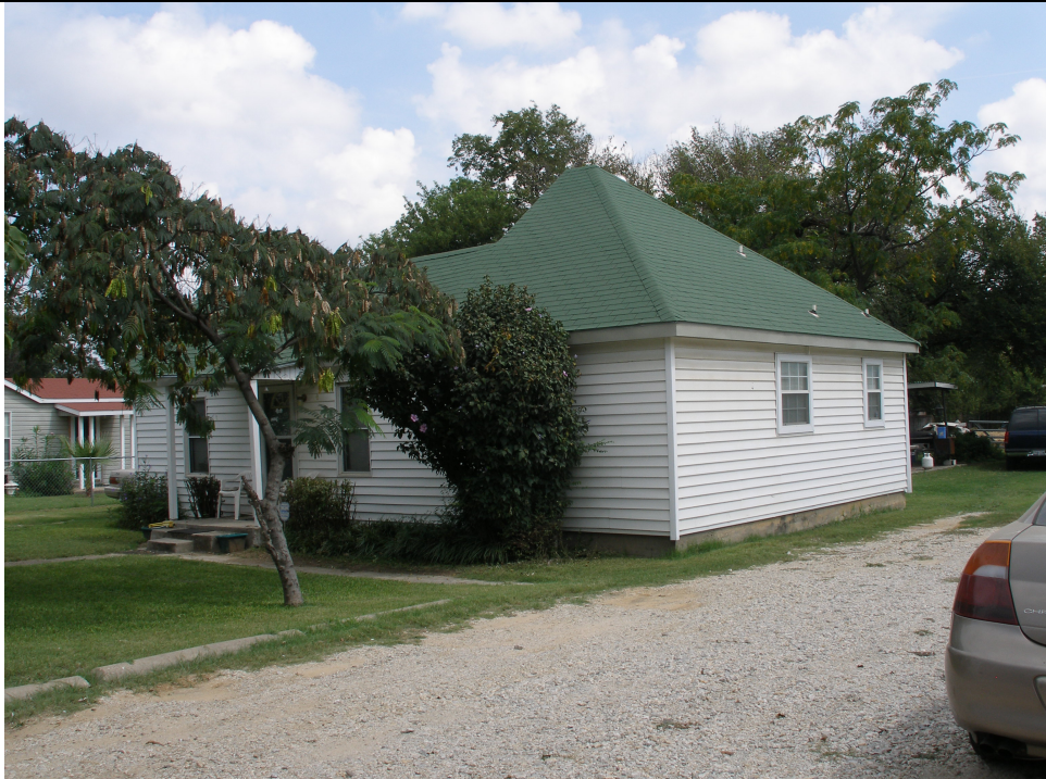
Resource Number 003, 1408 Carson Street, facing northeast.
