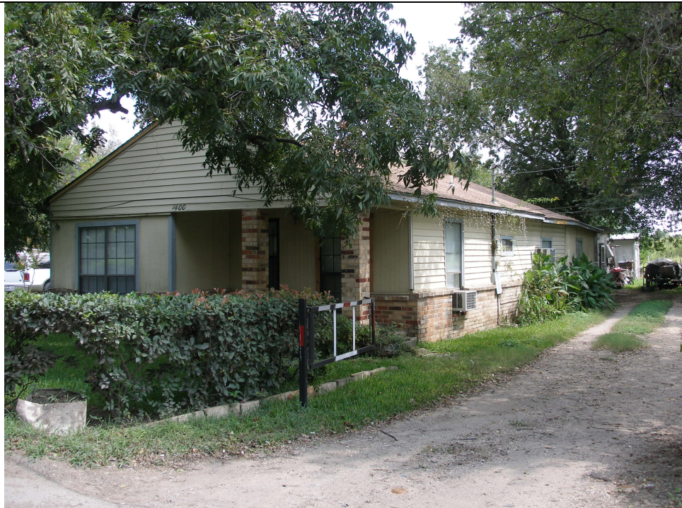
Resource Number 004, 1400 Carson Street, facing northeast.
