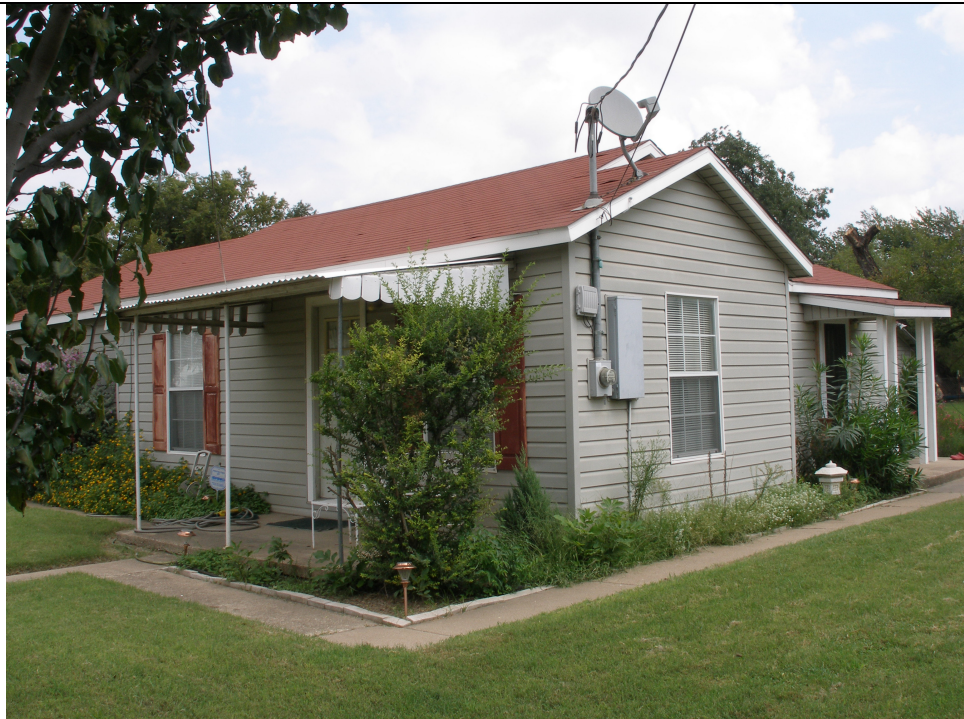
Resource Number 002, 1412 Carson Street, facing northeast.
