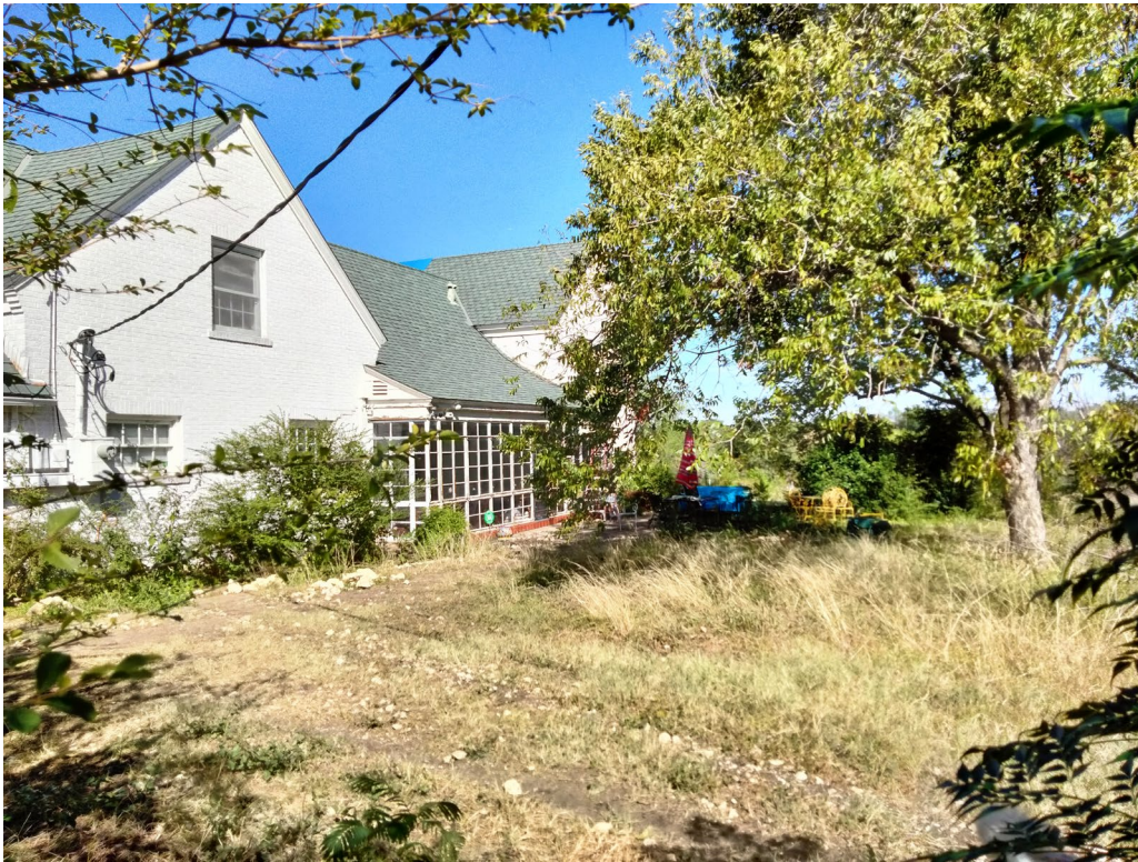
Fig. 8 – Showing the rear elevation and enclosed sunroom.
