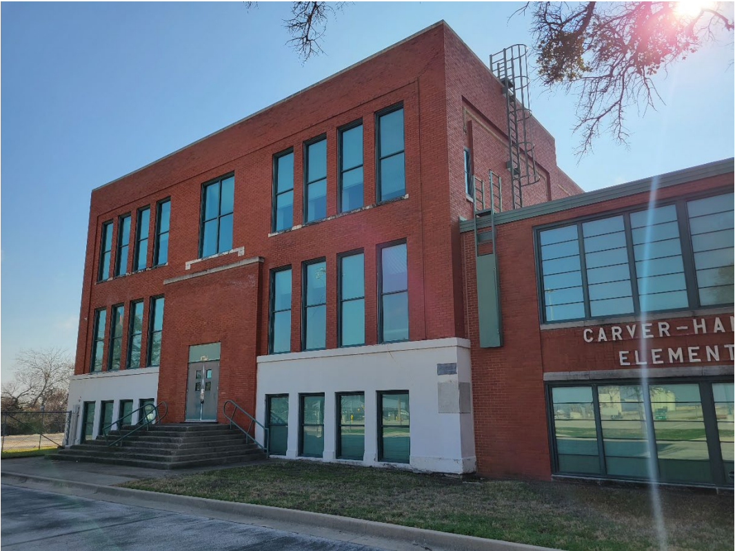
Figure 11 View of north facade
