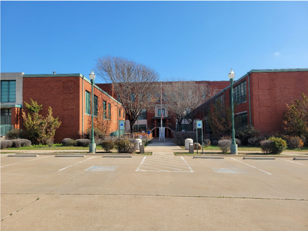
Figure 9 Front view of 1201 E 13 th St
