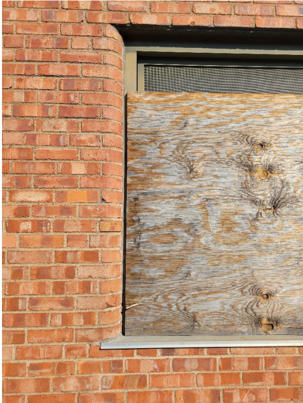
Figure 17 Detail view of curved brick at window; note replacement window materials
