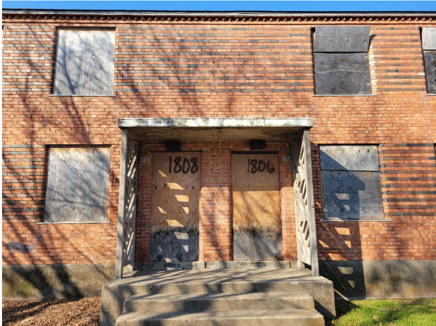
Figure 15 View entryway for 1801-1825 Stephenson St
