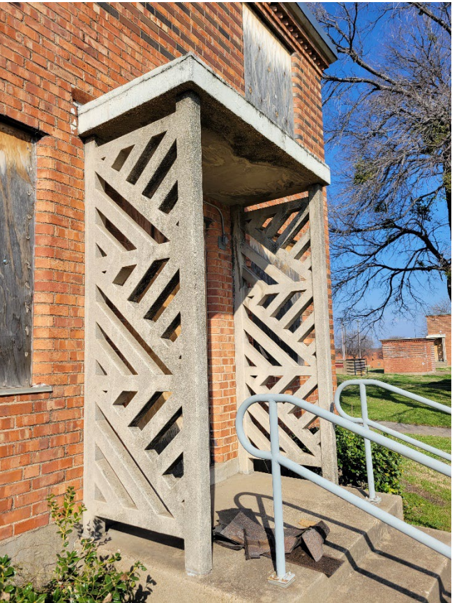
Figure 13 Cast Concrete porch supports
