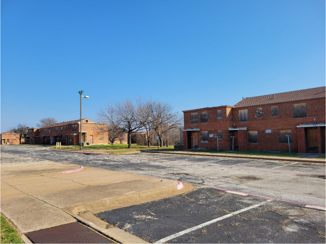
Figure 9 View of 1715-1750 (left) and 1801-1825 Stephenson St (right)
