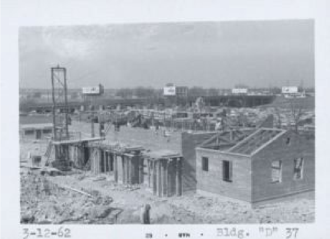
Figure 8 Construction of Butler Place additions; c. 1962
