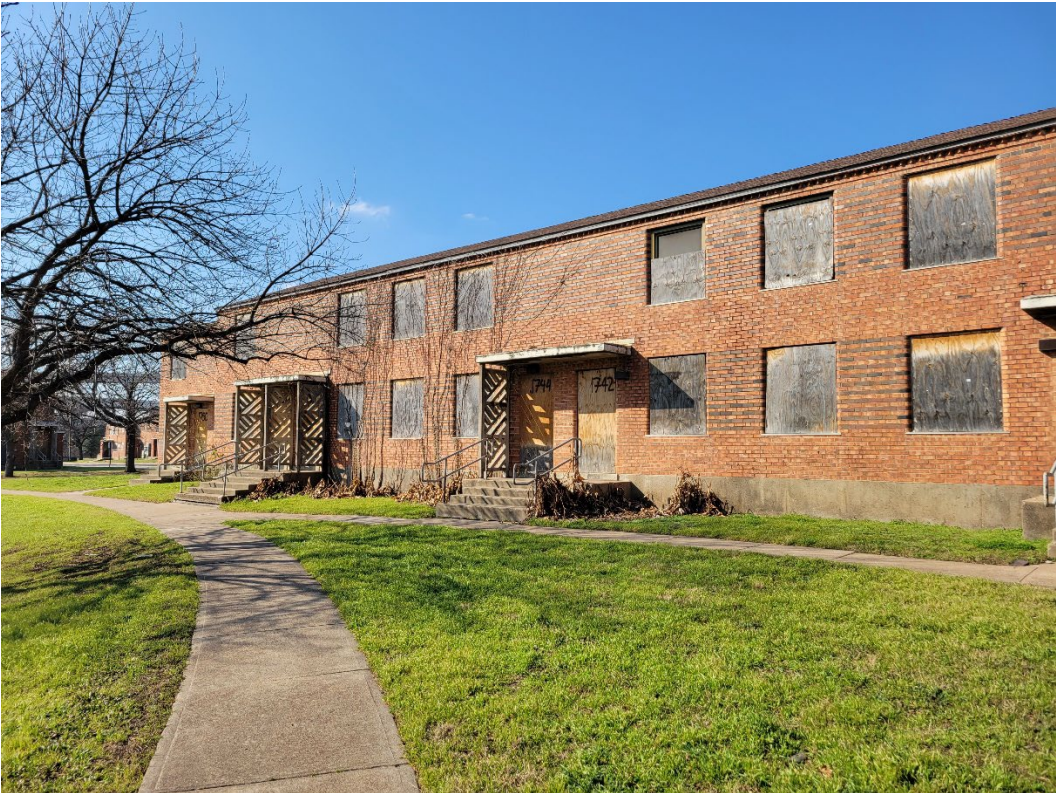
Figure 12 Rear view of 1715-1750 Stephenson St
