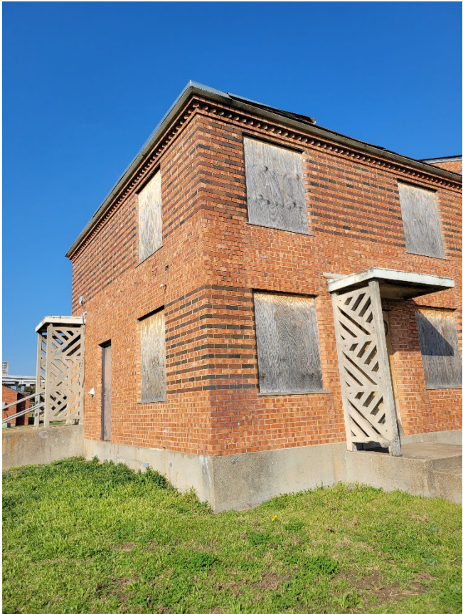
Figure 14 Corner view 1801-1825 Stephenson St
