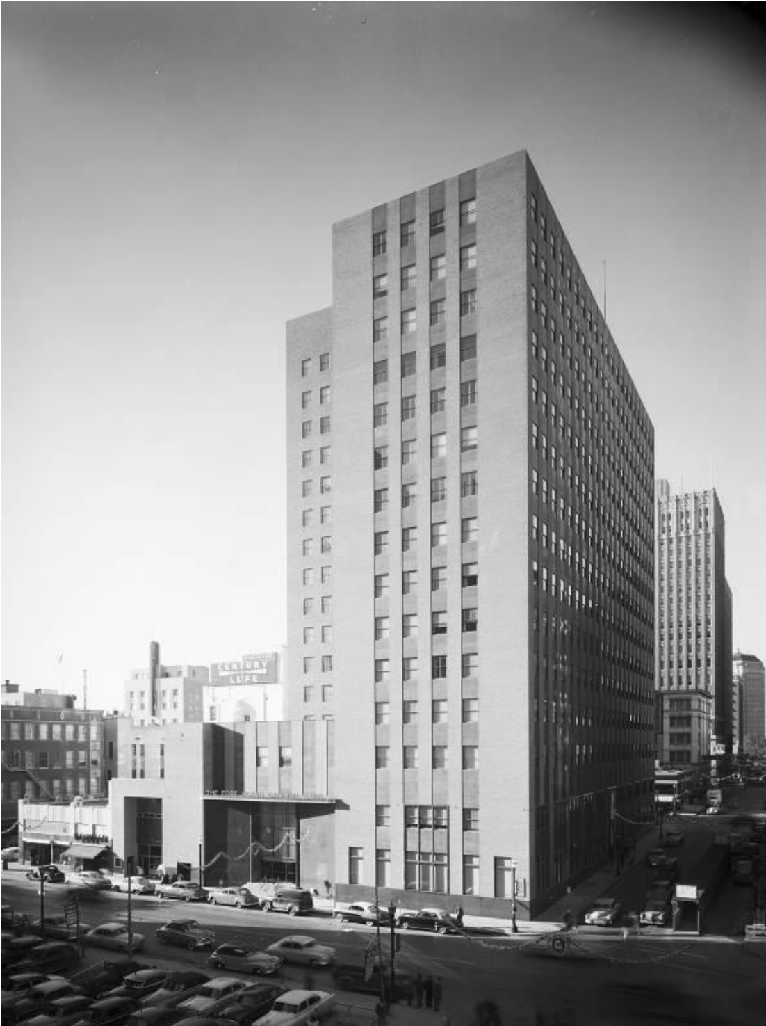
Figure 18: Exterior of Fort Worth National Bank Building, 1952. East elevation, looking southwest. Courtesy, W. D. Smith Commercial Photography, Inc. Collection, Special Collections, The University of Texas at Arlington Libraries. AR430-52-3-29. Identifier 20097271.
