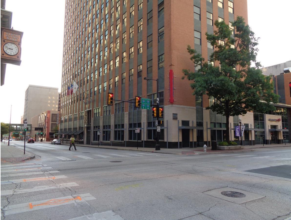
Photo 5: North and west elevations; looking southeast.
