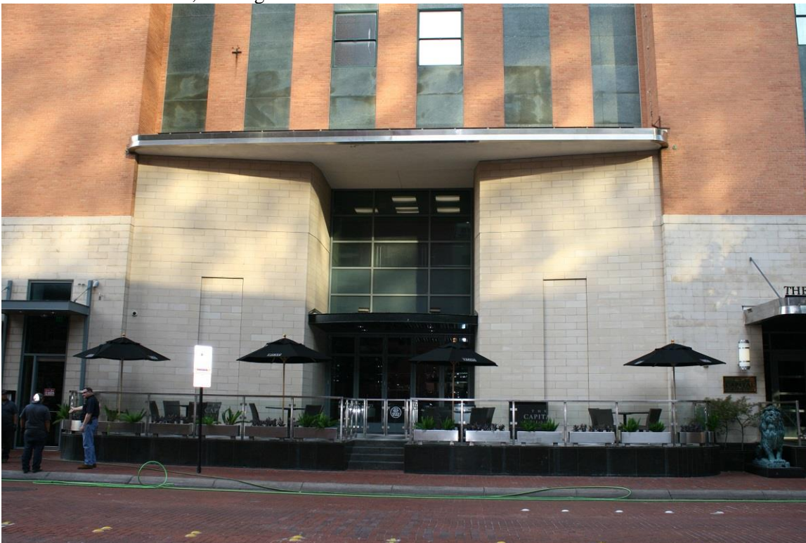
Photo 8: East entrance; looking west.
