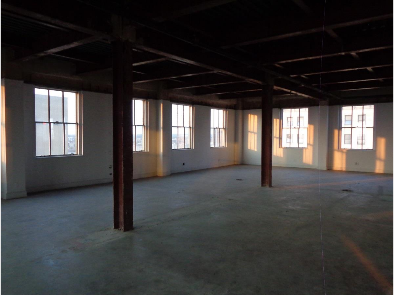
Photo 29: Sixteenth floor penthouse; looking southwest.
