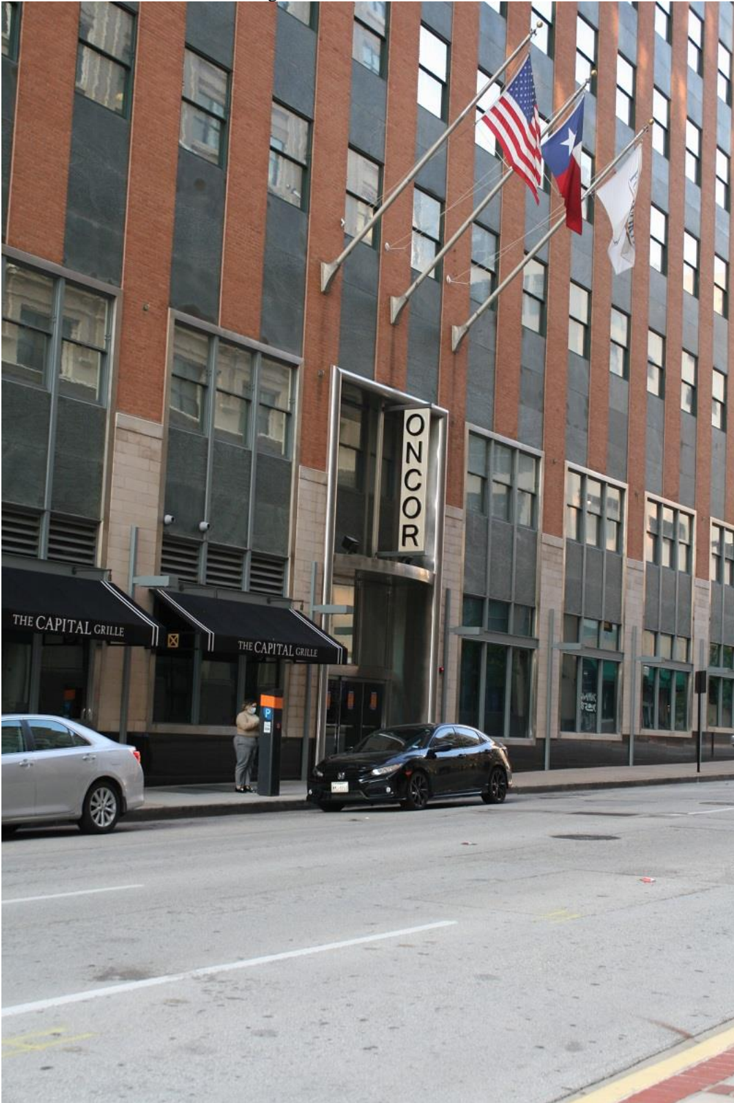
Photo 4: North elevation; looking southwest.
