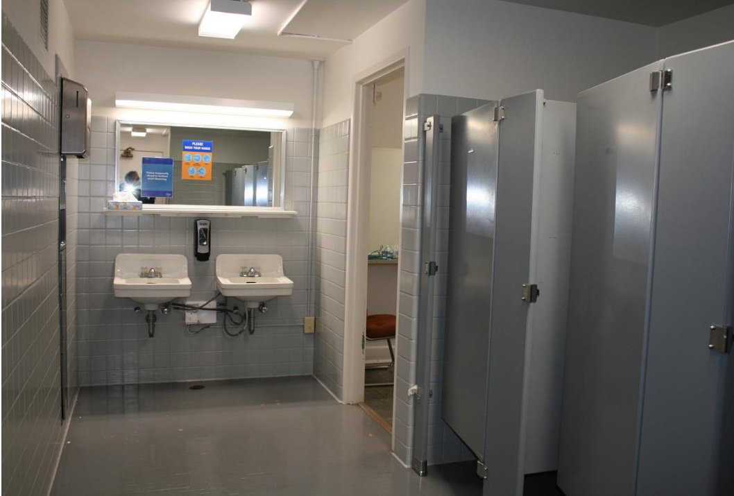
Photo 24: Fourth floor, women's restroom; looking south.
