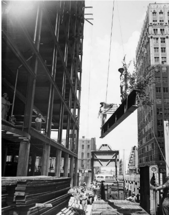
Figure 15 Fort Worth National Bank, 07/31/1951. H. Warren Smith, steel foreman, and Ed Grimes, inspector, ride the beam as the last piece of steel is hoisted into position atop the new Fort Worth National Bank Building. Courtesy, Fort Worth Star-Telegram Collection, Special Collections, The University of Texas at Arlington Libraries. AR406-6-457. Identifier 20126776.
