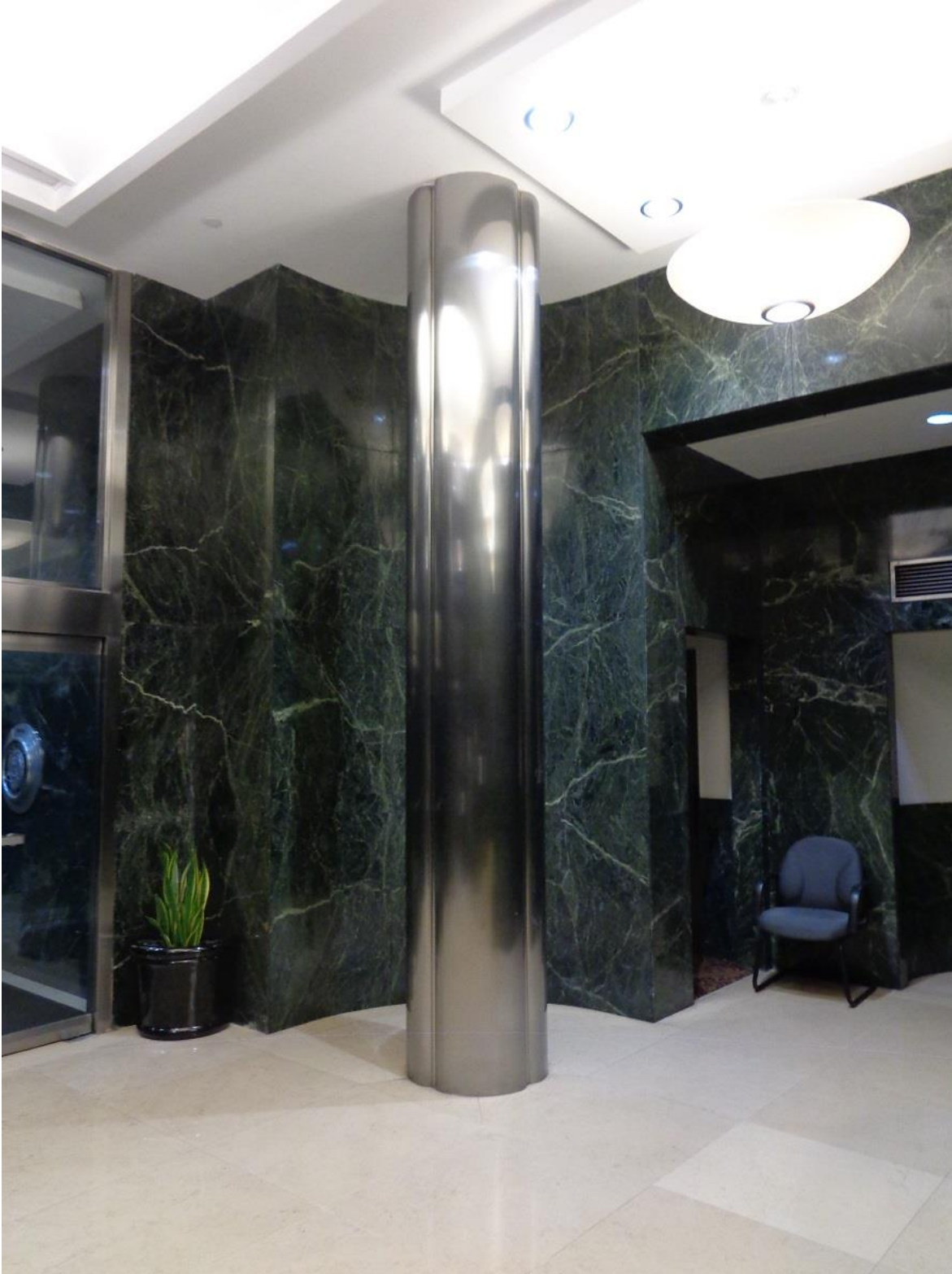
Photo 16: Stainless steel column and Maryland Verde Antique stone in first floor elevator lobby; looking northeast.
