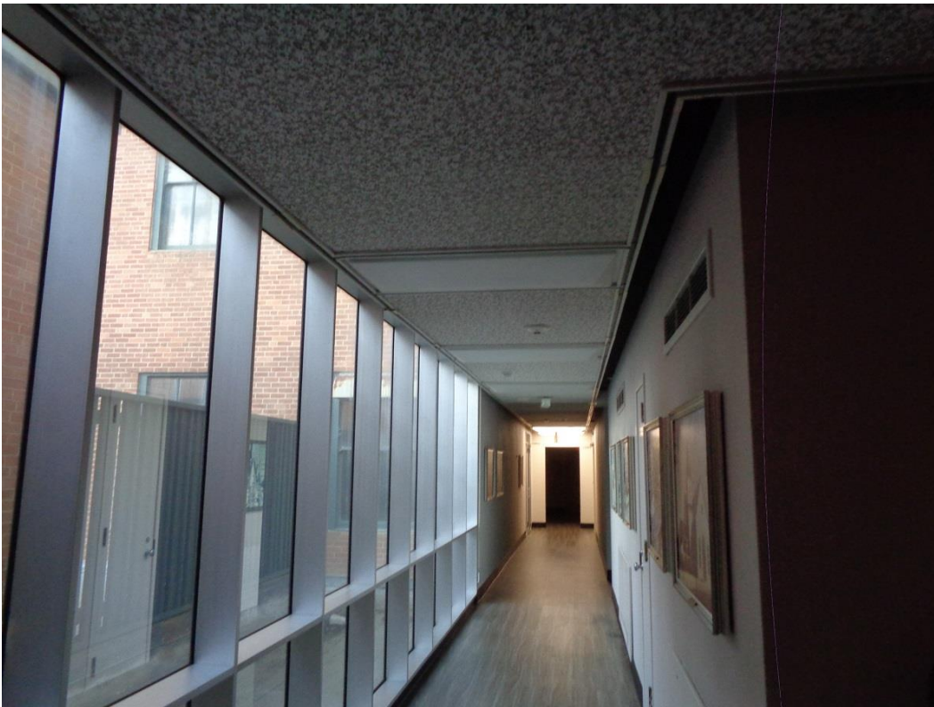
Photo 25: Fourth floor lightwell; looking west.
