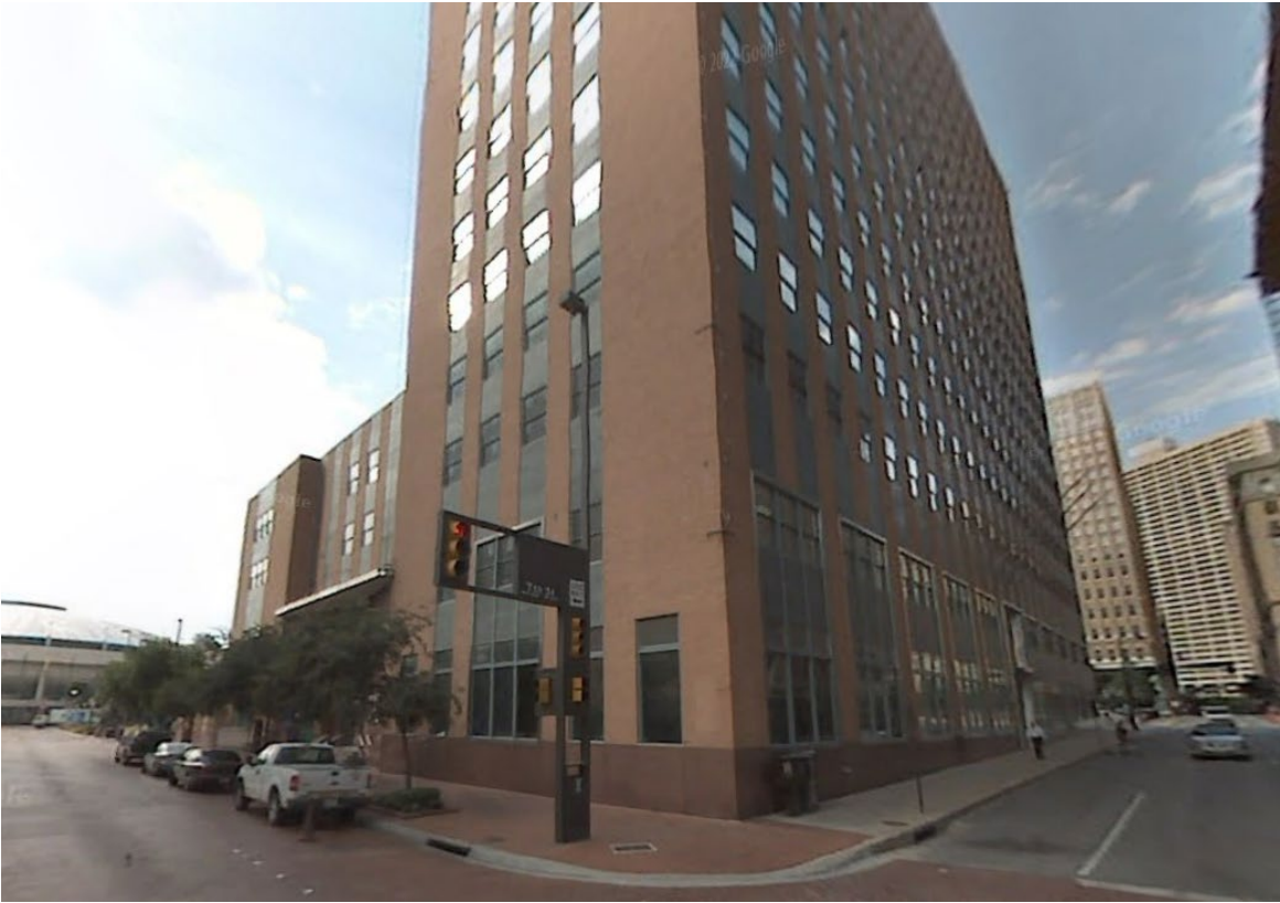
Figure 5 Google Street View of 115 W 7 th St circa 2007 before the 2011 exterior renovations to the first and second floors. NEC at 7 th and Main St.
