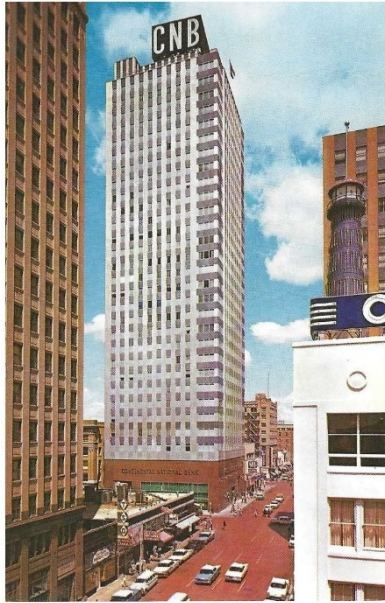
Figure 26 Continental National Bank Building, West 7th and Houston Streets. Designed by Preston M. Geren, Architect and Engineer (1952, 1956-57, demolished 2006). View looking north up Houston Street. Fort Worth National Bank Building is in the background, right side of the photograph. Strykers' Western Fotocolor, Artist Photographers, Fort Worth, Texas (authors' collection).
