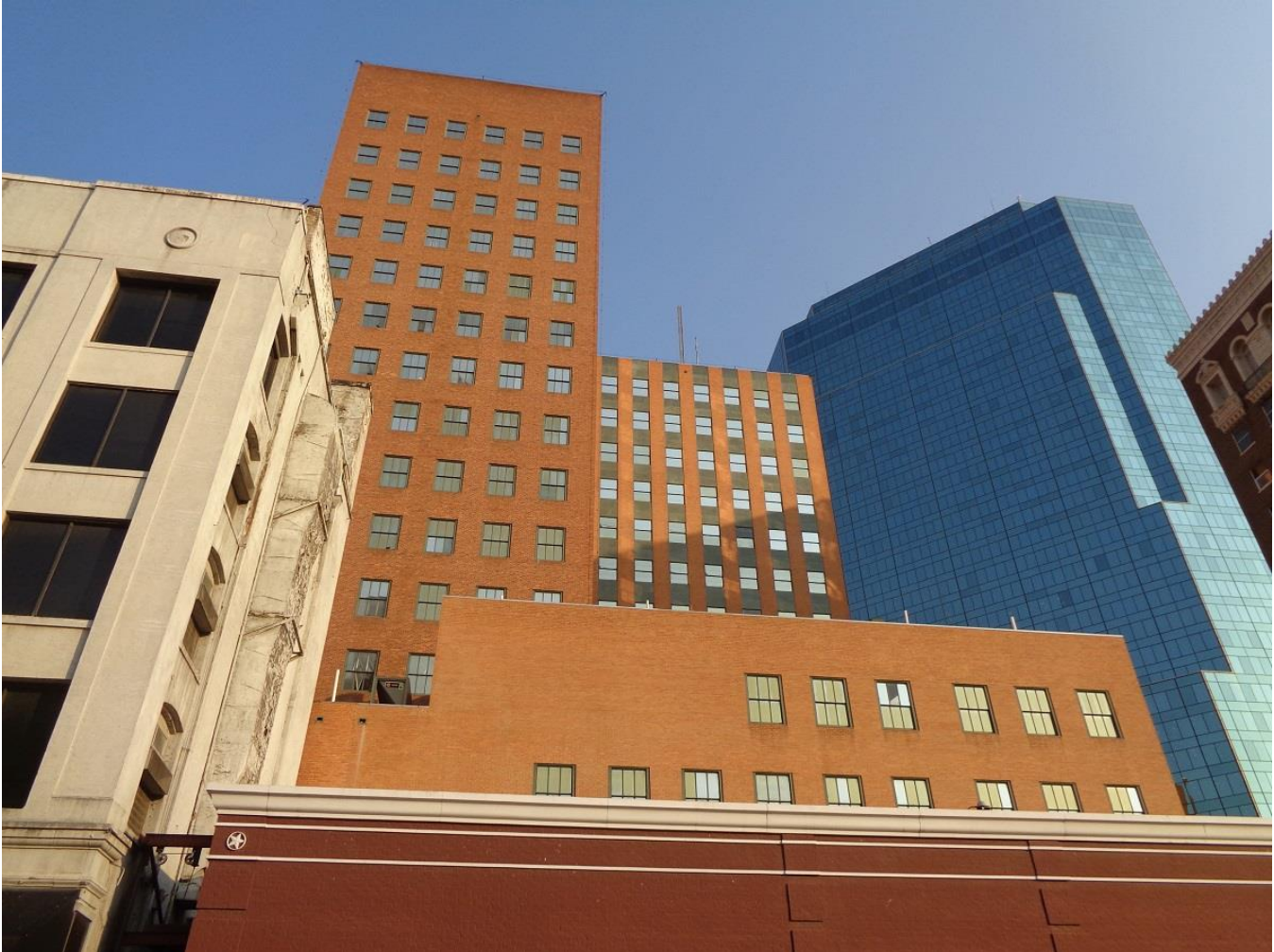
Photo 10: South elevations of tower, base, and slab; looking north.
