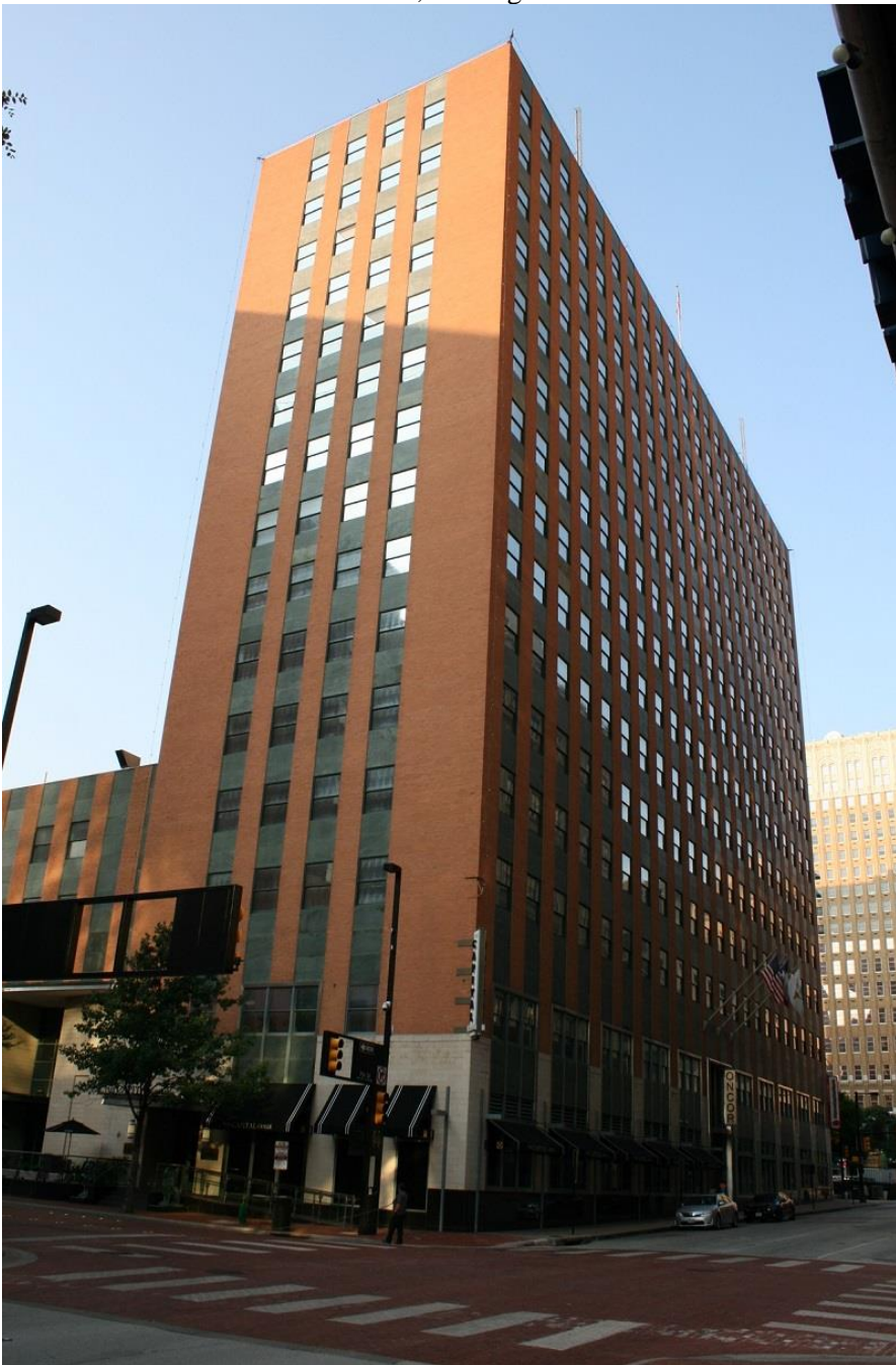
Photo 1: East and north elevations; looking west.
