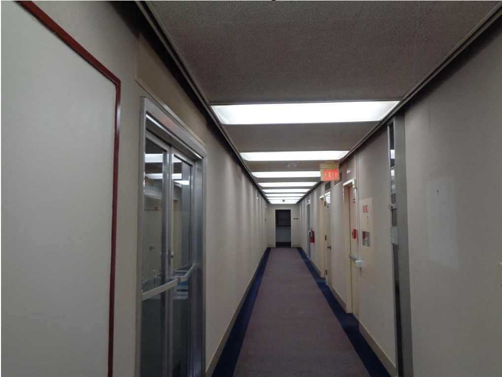
Photo 27: Tenth floor historic corridor; looking east.
