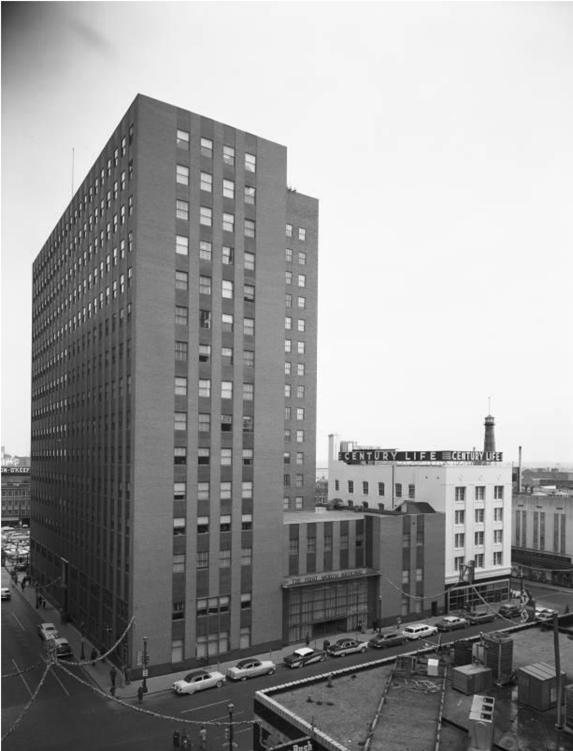
Figure 20: Exterior of Fort Worth National Bank Building, 1958. West elevation, looking southeast. Courtesy, W. D. Smith Commercial Photography, Inc. Collection, Special Collections, The University of Texas at Arlington Libraries. AR430-58-1-150. Identifier 20191685.
