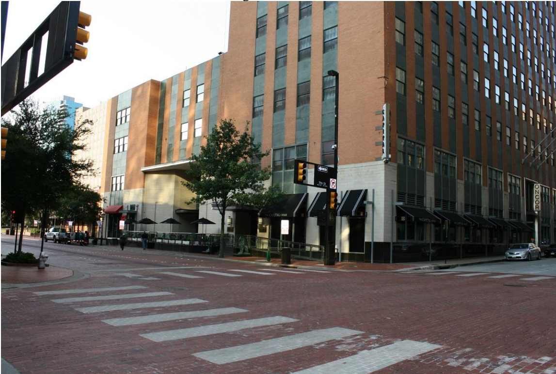
Photo 7: East and north elevations; looking southwest.
