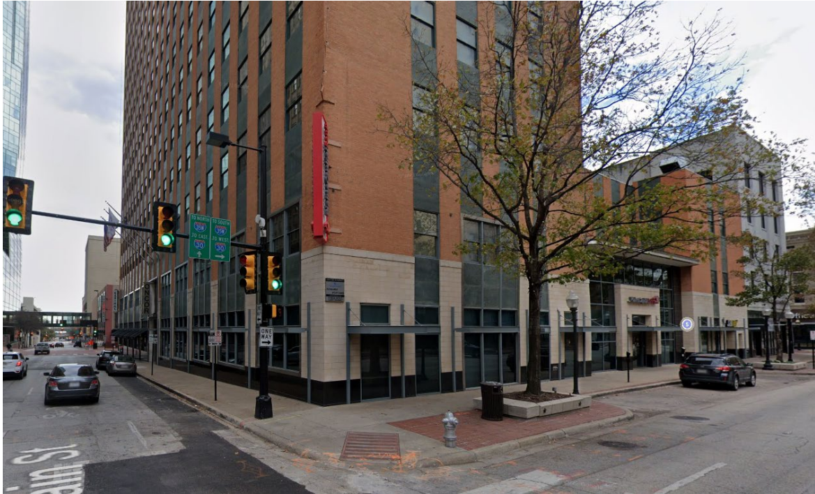
Figure 4 Google Street View of 115 W 7 th St circa 2022 after the 2011 exterior renovations to the first and second floors. NWC at 7 th and Houston. Note the awnings, additional storefront windows, and material changes.
