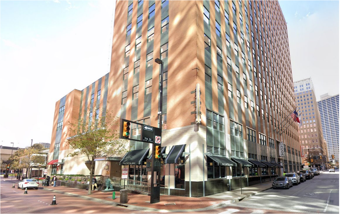
Figure 6 Google Street View of 115 W 7 th St circa 2022 after the 2011 exterior renovations to the first and second floors. NWC at 7 th and Houston. Note the awnings, Oncor signage, additional storefront windows, material changes, ramp and outdoor patio area for a restaurant tenant.
