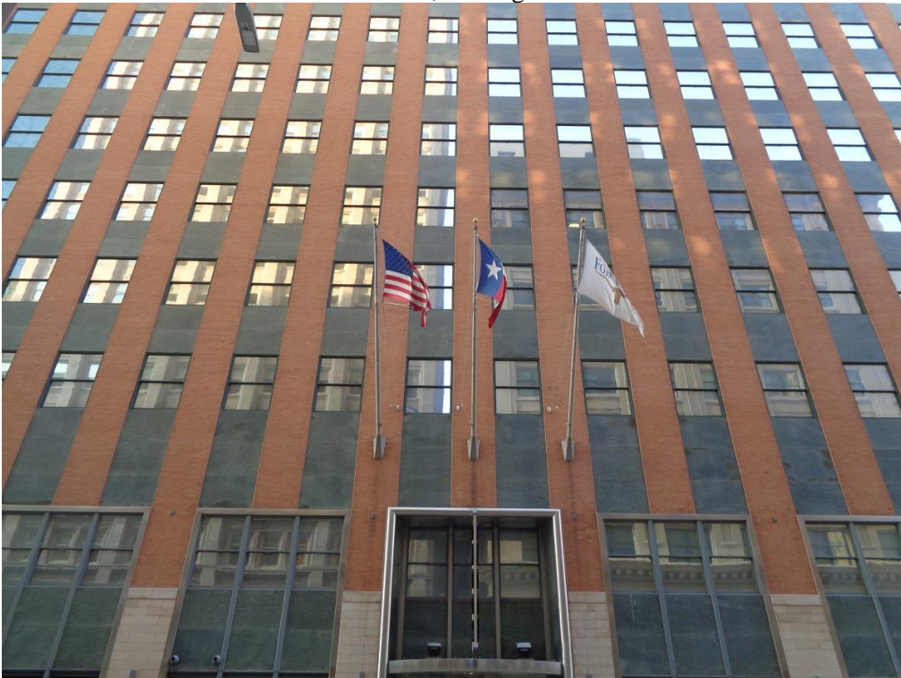
Photo 6: North elevation above entrance; looking south.
