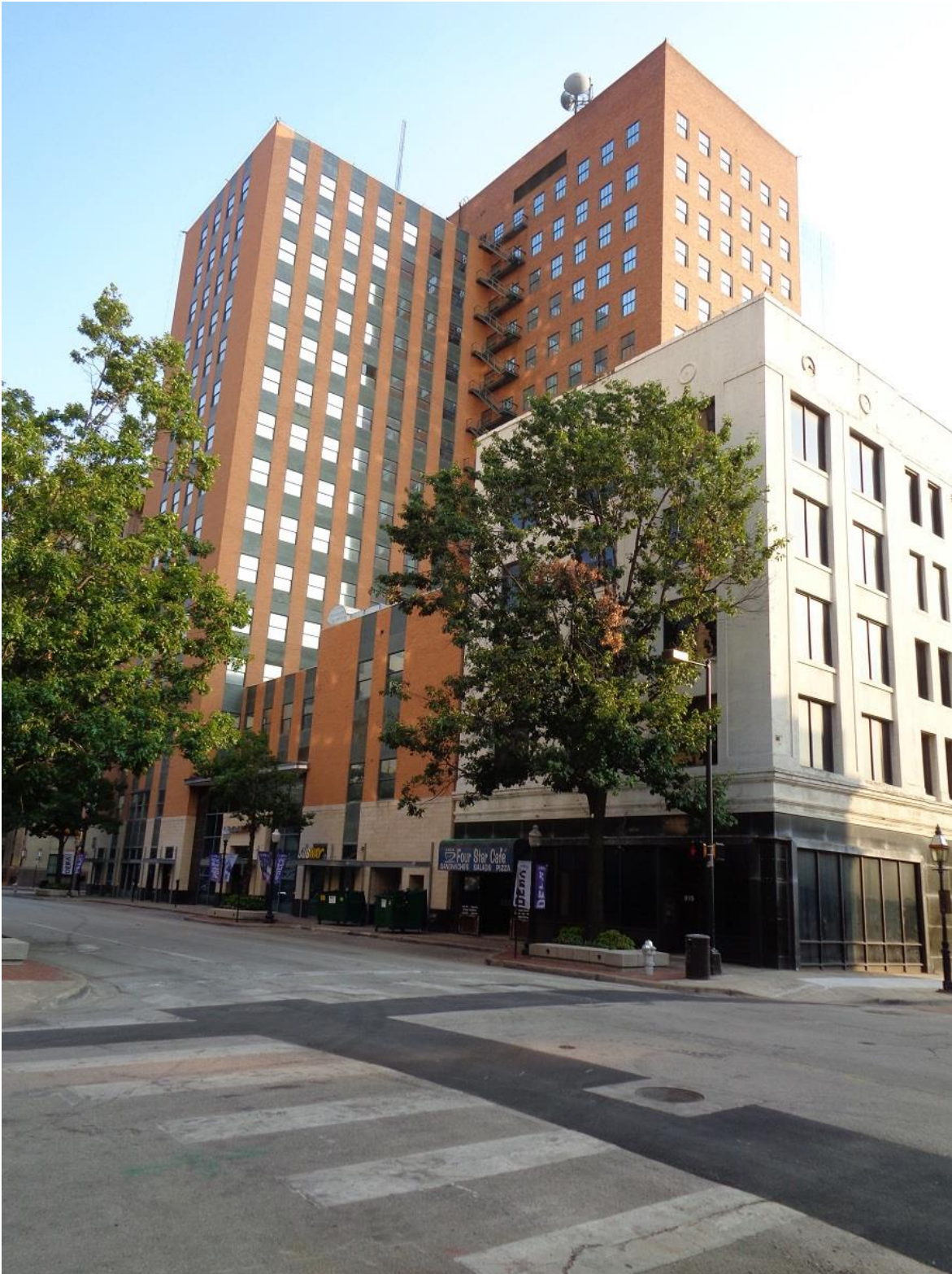
Photo 11: West and south elevations, slab, base, and tower; looking northeast.
