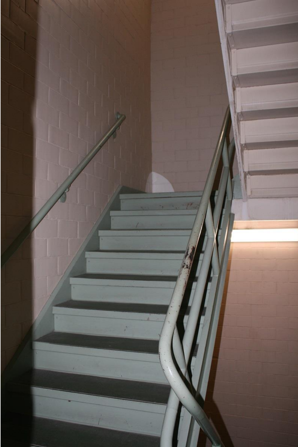
Photo 23: Fourth floor, west stairs; looking south.
