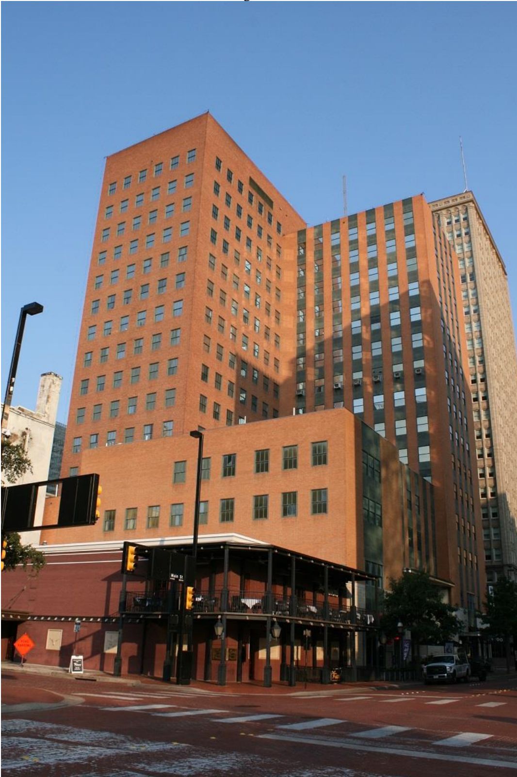
Photo 9: South and east elevations; looking northwest.
