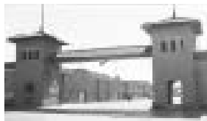
The entrance to the Horse and Mule Barns is marked by two two-story towers, each with round arched openings at the base and three small round arched openings on the second level.
