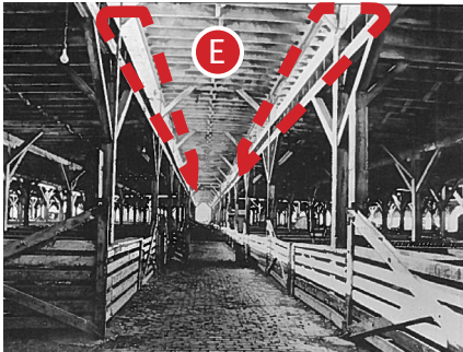
Early hog & sheep barns and pens were roofed with a “Y” frame construction with clerestories for sunlight and air flow (E).
