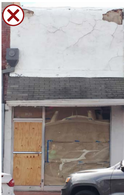
Before: Historic material covered
