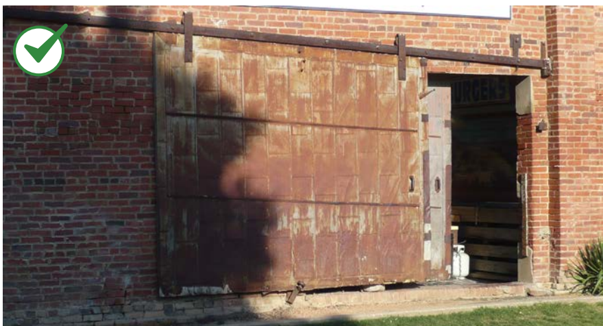
Preserve historic doors and their openings.
