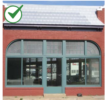
Retain historic coatings such as paint that help protect exterior materials from moisture and ultraviolet light.
