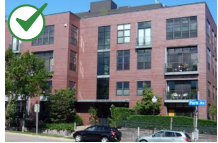
Use vertical and horizontal articulation design techniques to reduce the apparent scale of a larger building mass.
