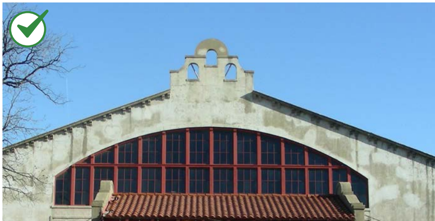
Use special care when replacing a window on a primary facade.
