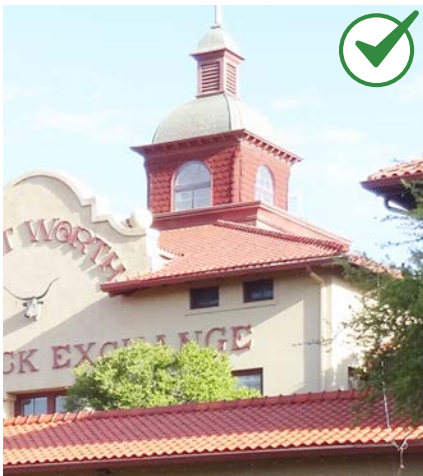
Use replacement roof materials that are similar in scale, texture, finish and color to traditional roof materials.
