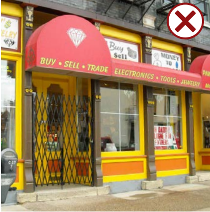
Do not install curved form awnings on a rectangular opening or use colors that are not compatible with the structure.
