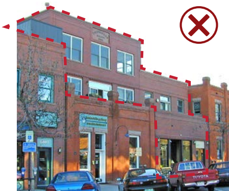
This three-story roof addition and side addition overwhelms the historic building due to its disproportion in mass and scale.
