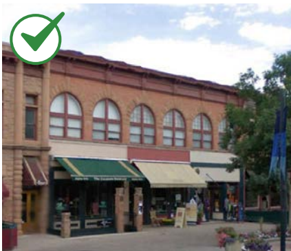
The removal of the inappropriate garage door and the rehabilitation of this commercial building successfully returns the property to the state that preserves the building's historic integrity.
