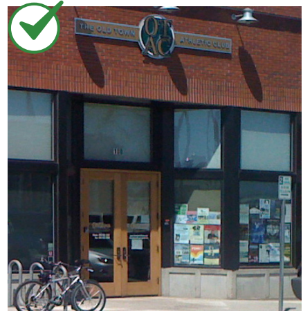
A simplified or contemporary interpretation of a traditional storefront may be considered where the historic storefront is missing and no evidence of it exists.
