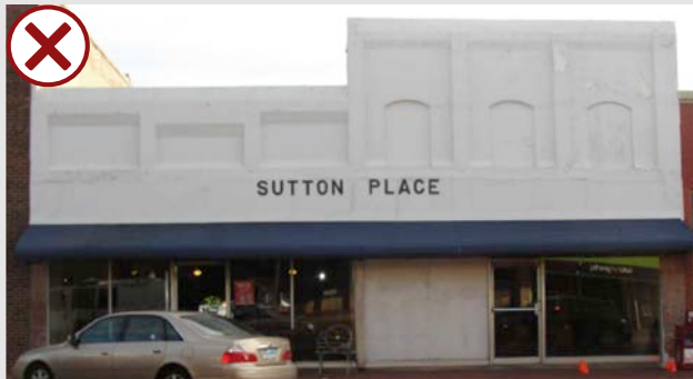
Before: moderately altered historic building
