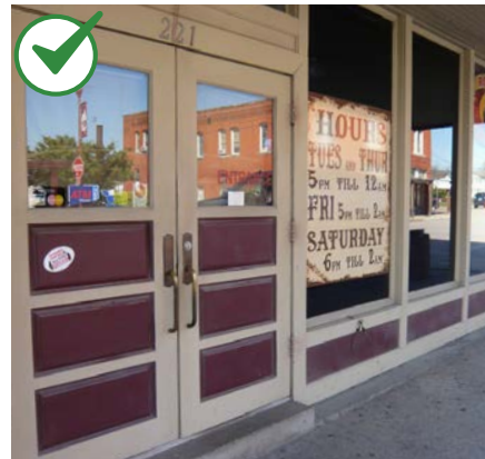
Preserve historic and decorative features including door frames, sills, heads, jambs, moldings, detailing, transoms and flanking sidelights.
