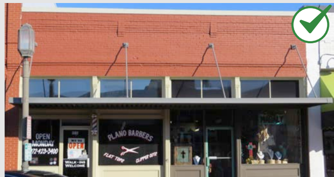
After: rehabilitation includes a reconstructed historic storefront, a historically accurate canopy and exposed original materials
