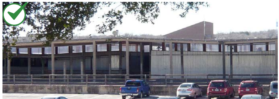
Maintain the original roof line and shape on a historic structure. The roof of the Stockyards Station building (the historic sheep and hog pen area) is a distinctive feature that should be preserved.
