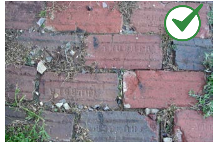
Historic paving materials, such as brick, should be preserved and maintained.
