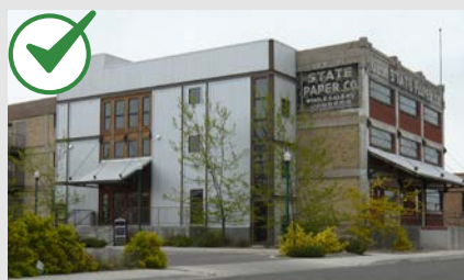
An addition, located along a secondary wall retains the ability to perceive the historic character of the building.
