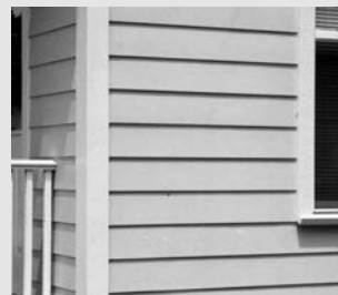
Fiber cement siding
