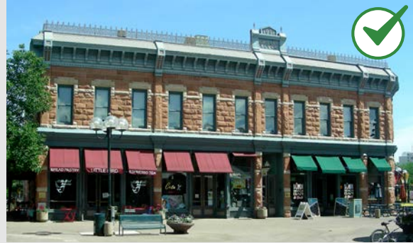
After: Original storefronts revealed.
