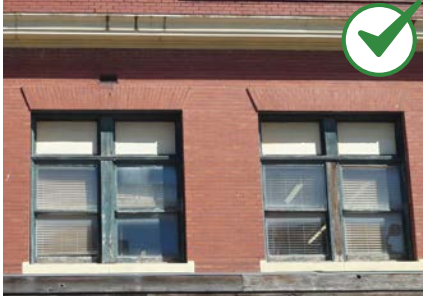
Repair, rather than replace, frames and sashes.
