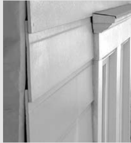
Fiber cement siding
