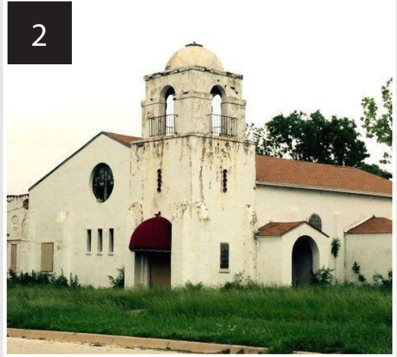
Once scheduled for demolition the building was not maintained and was left abandoned and dilapidated.
