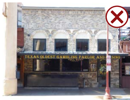
Many historic features, including the window openings and storefront, have been substantially altered on this property.
