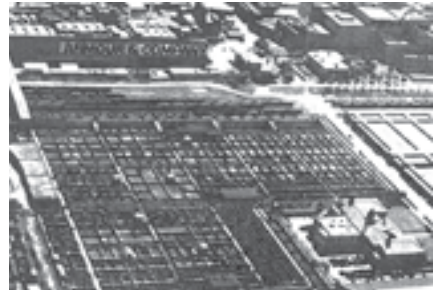
Buildings at the two meat packing plants step down in scale along the eastern edge (M).
