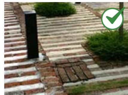
Reuse historic paving material to define outdoor use areas.
