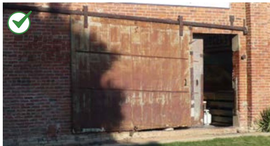
Preserve historic doors and their openings.
