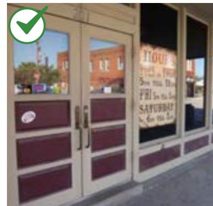
Preserve historic and decorative features including door frames, sills, heads, jambs, moldings, detailing, transoms and flanking sidelights.
