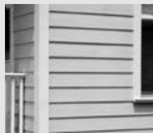
Fiber cement siding
