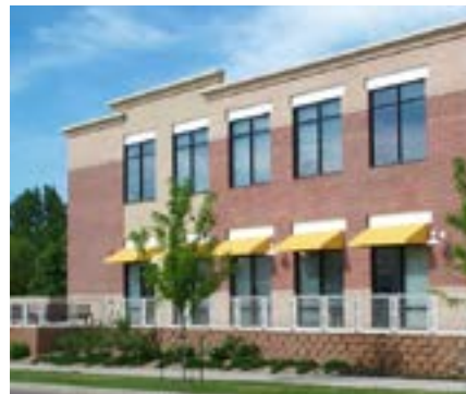
» Treatment of a side, or secondary wall: » Horizontal articulation (change in material) » Masonry » Vertical articulation (wall offset) » Landscaped edge
