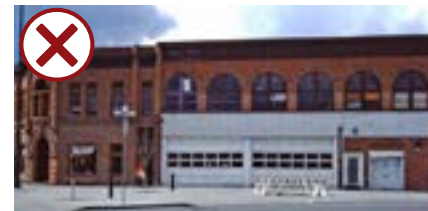
A change in use that requires alteration of key features, such as this, should be avoided.
