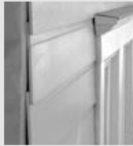
Fiber cement siding
