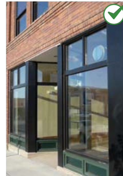
Use high quality design and depth of detail in building features to enhance compatibility with the historic context.
