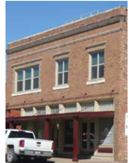
This example of a recently rehabilitated building shows a contemporary entry to the historic facade.
