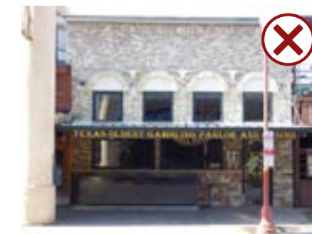
Many historic features, including the window openings and storefront, have been substantially altered on this property.
