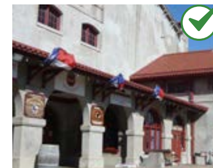
Protect and maintain historic stucco.
