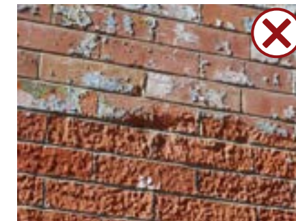
Do not use harsh cleaning methods, which can inhibit the function and/or appearance of the historic material, (such as sandblasting, which can damage its protective coating).
