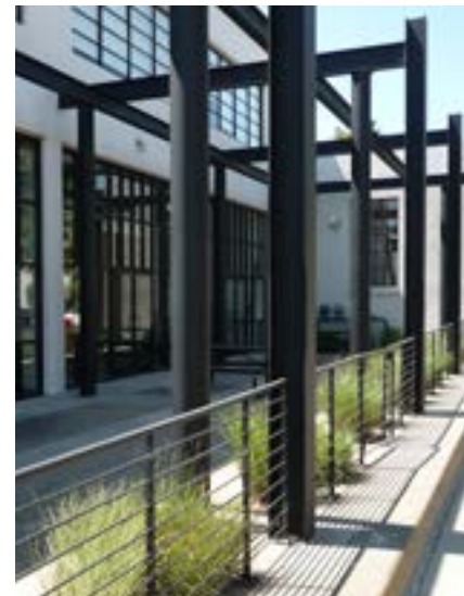
Landscaped areas that can be enjoyed, both visually and functionally, should be provided in a project when feasible.
