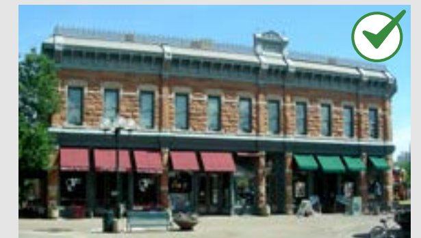
After: Original storefronts revealed.
