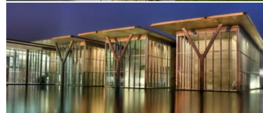
Innovative new designs that draw upon regional design traditions are preferred. These example buildings incorporate timber framing that resembles the construction of the pen areas in the Stockyards.
