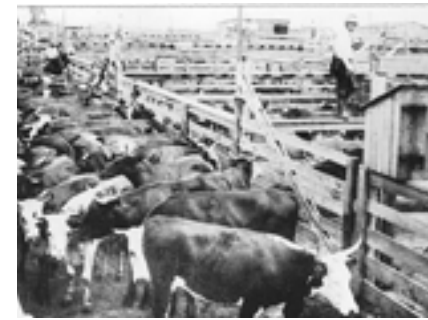
Cattle pen area showing wood and steel gusset fencing.
