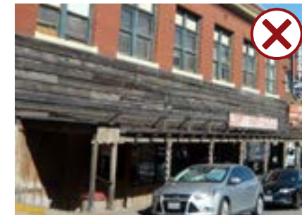
If the original transom glass is missing, installing new glass is preferred. If a transom must be blocked out, be certain to retain the original proportions and framing divisions.
