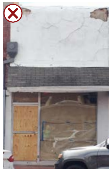
Before: Historic material covered
