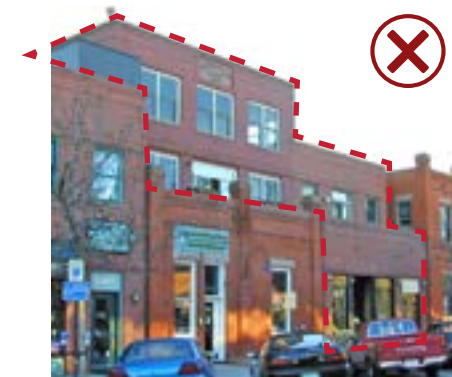
This three-story roof addition and side addition overwhelms the historic building due to its disproportion in mass and scale.
