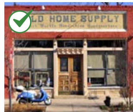
Use a color scheme that is compatible with the historic character of the structure.
