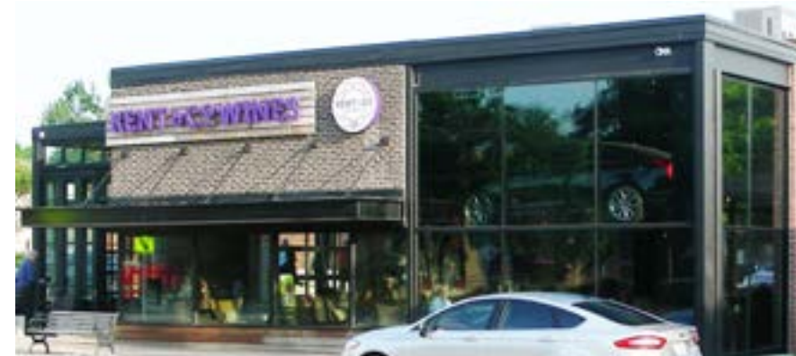
» Street level activation (shopfront)
