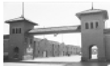
The entrance to the Horse and Mule Barns is marked by two two-story towers, each with round arched openings at the base and three small round arched openings on the second level.
