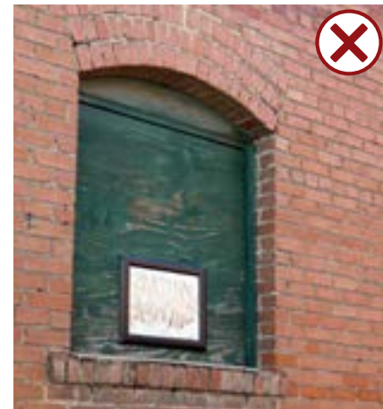
Restore a historic window opening that has been altered. For example, this opening has been blocked. Restoring the window is best practice in this situation.
