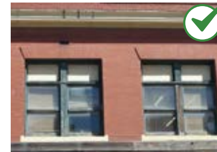
Repair, rather than replace, frames and sashes.
