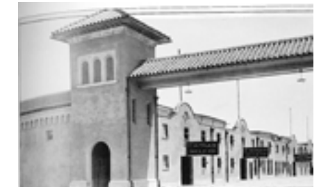
View of the east entry tower that frames Horse and Mule Alley. The eastern Horse and Mule Barns can be seen in the background.
