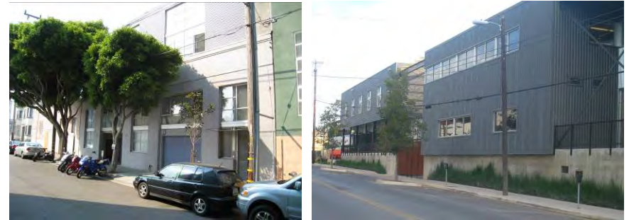
Appropriate design and character of industrial buildings
