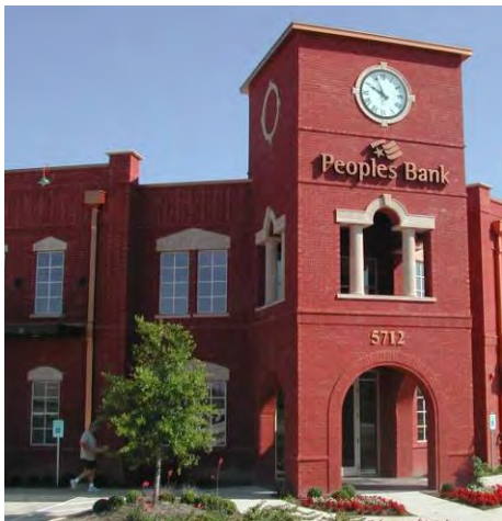
Tower element at a corner
