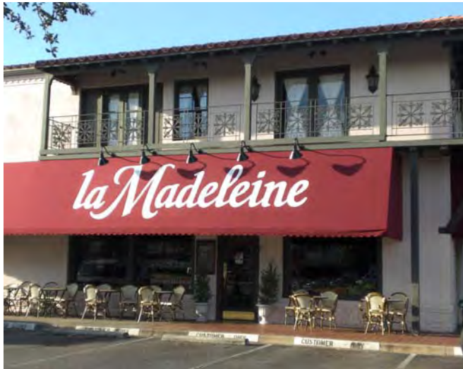
Typical storefront with a façade rhythm of approximately 20’
