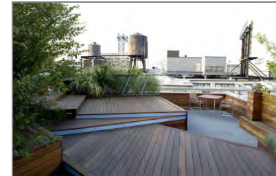
Image of a roof terrace
