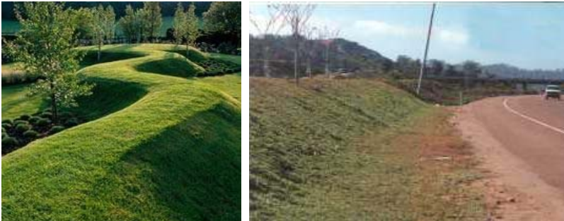
EXAMPLES DO NOT EXPRESS A NATURAL VERTICAL CHANGE IN ELEVATION OVER THE LENGTH OF THE BERM
