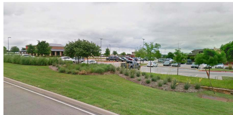
Fig. 23.2 Examples of compliant landscape screening
