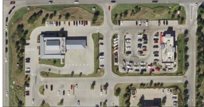
Fig. 22.2 Example of width changes along landscape earthen berms
