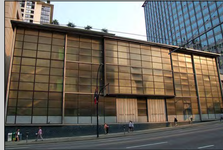
Both photographs represent creative ways to screen utilitarian requirements in any city such as power substations
