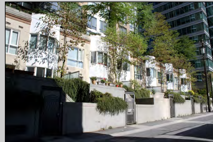
Privacy fence for residential units
