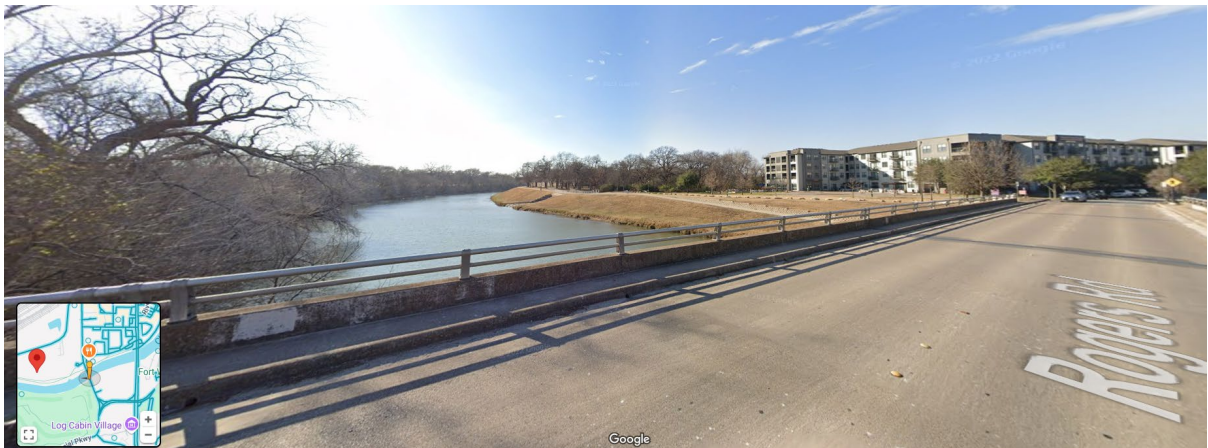
Figure 5 Google Street View looking at the subject property from the Rogers Road bridge. The apartments on the right are 4 stories.
