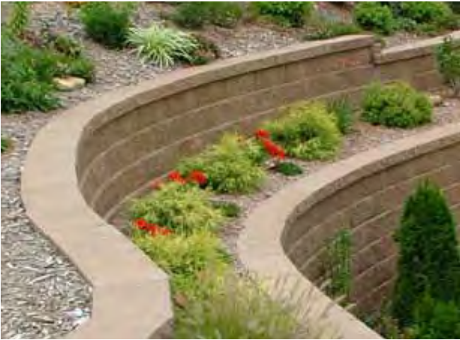
8.11.2.A1: Example of terraced retaining wall
