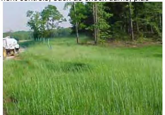
Figure 7.10-16: Vegetated Filter Strip
