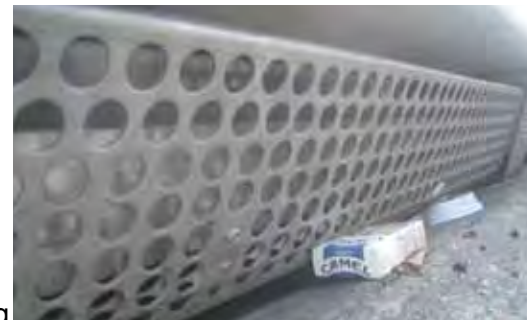
Figure 7.10-18: Catch Basin Opening Cover
