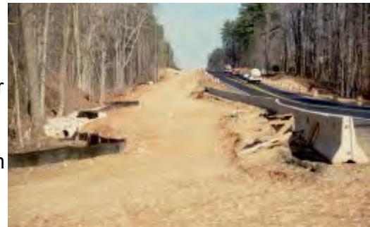
Figure 7.10-14: Temporary Mulch and Seeding
