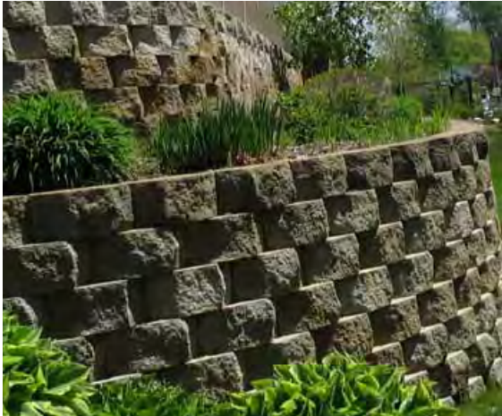
8.11.2.A5: Masonry retaining wall
