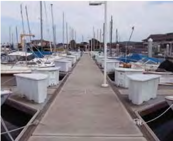
8.11.4.D3: Main walkway
