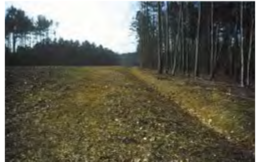
Figure 7.10-5: Temporary Silt Ditch
