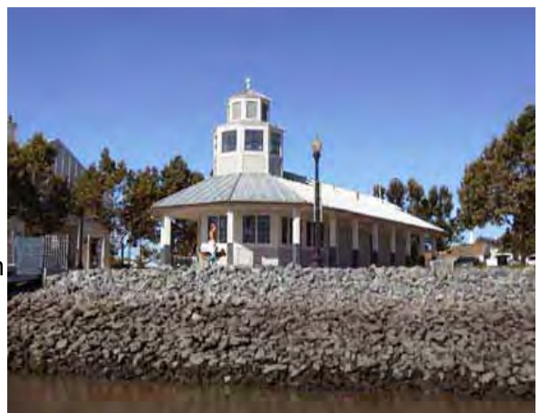
8.11.4.H4: Restroom facility
