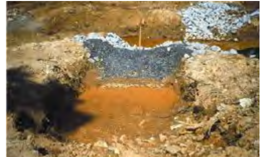
Figure 7.10-7: Temporary Rock Sediment Dam
