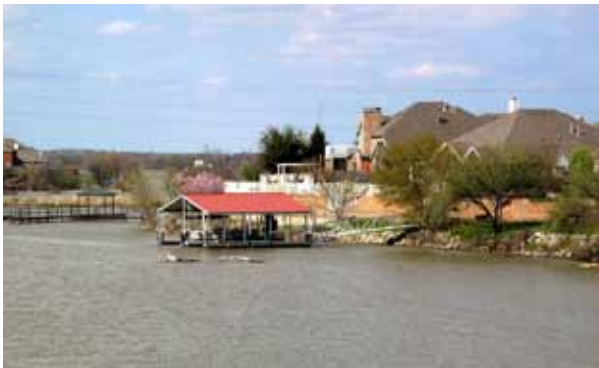
Single family development at southern end of lake
