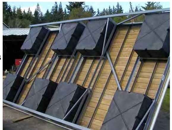
8.11.3.F3: Encased flotation material
