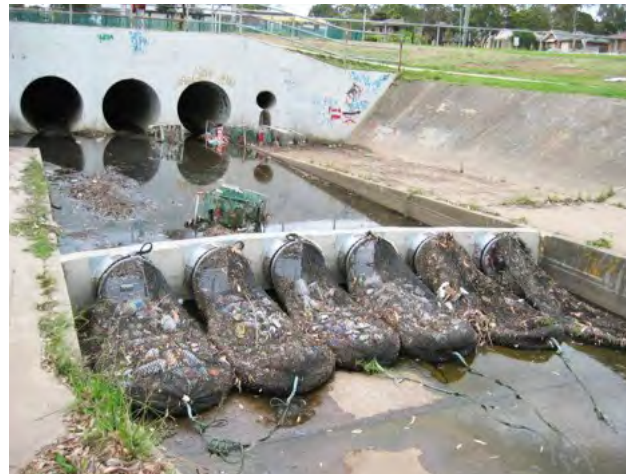
Figure 7.10-21 End-of-pipe Netting Device
