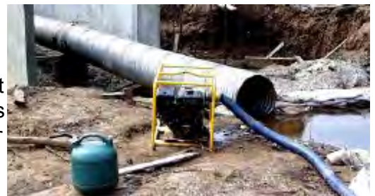
Figure 7.10-8: Piped Diversion
