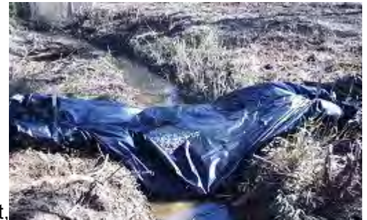
Figure 7.10-410: Stone with Impervious Fabric
