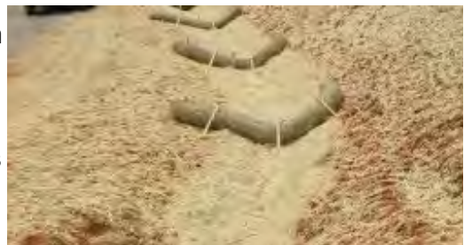
Figure 7.10-6: Fiber Check Dam
