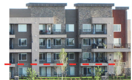
Distinction between the first and upper levels with balconies and material change
