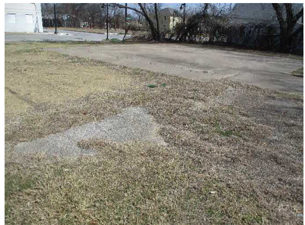
Photo #6 View of the concrete remnant foundation at 901 Evans Avenue.
