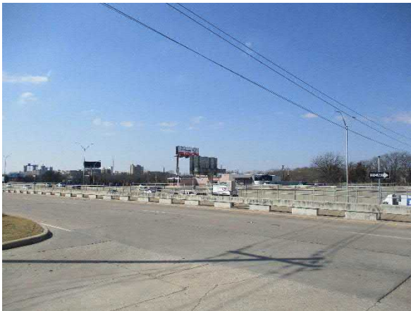
Photo #21 View of the western adjoining South Freeway, followed by I-35.
