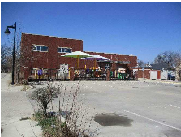
Photo #17 View of the eastern adjoining Bethlehem Community Center (920 Humbolt Street).
