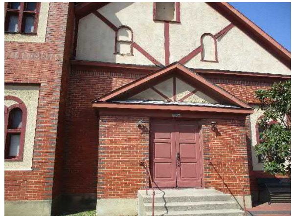
Photo #16 View of the southern adjoining Historical Sunshine Cumberland facility (1100 Evans Avenue).
