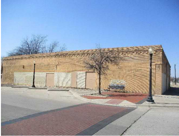
Photo #7 View of the vacant building located at 900 Evans Avenue.
