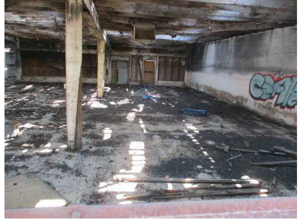
Photo #8 Interior view of the building located at 900 Evans Avenue.
