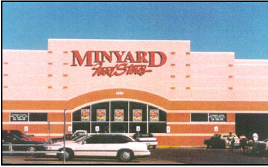
Through federal low interest loans, the City of Fort Worth encouraged Minyard Food Stores to invest over $11 million in Southeast Fort Worth. The new grocery store at the corner of Miller Drive and East Berry Street provide a much needed service to the surrounding community.
