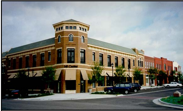
Corner buildings at the gateways to Evans & Rosedale can announce the block with a dominant architectural element.
