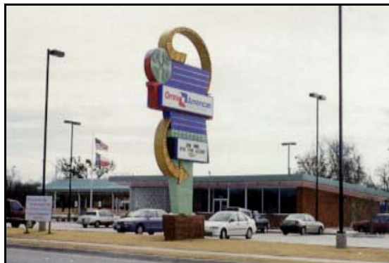
New business investment is occurring in Southeast Fort Worth. Omni America converted an old drive-in restaurant into a federal credit union at this East Rosedale site within one-half mile of Heritage Center.
