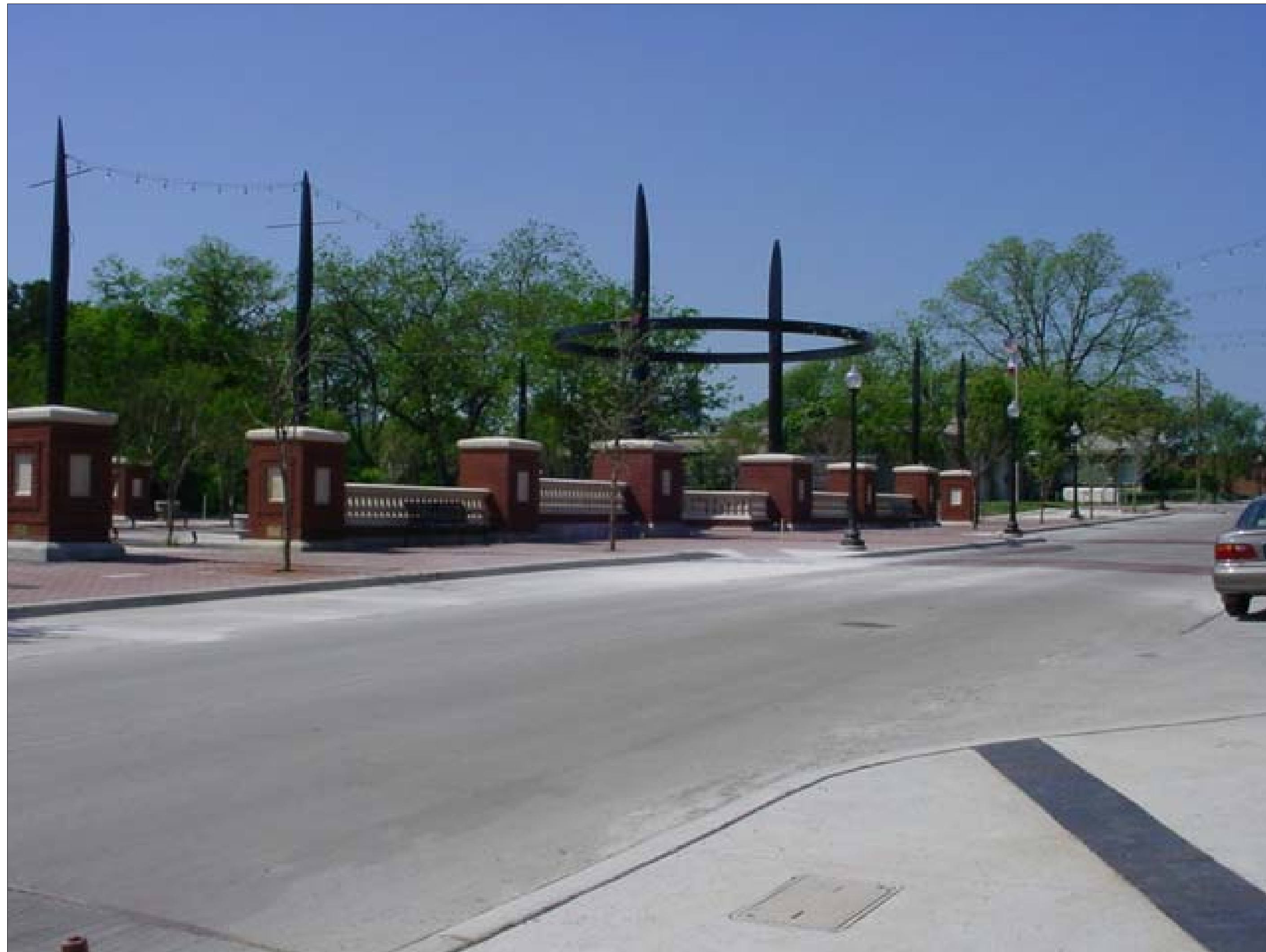
PLAZA VIEW FROM EVANS AVENUE LOOKING NORTH
