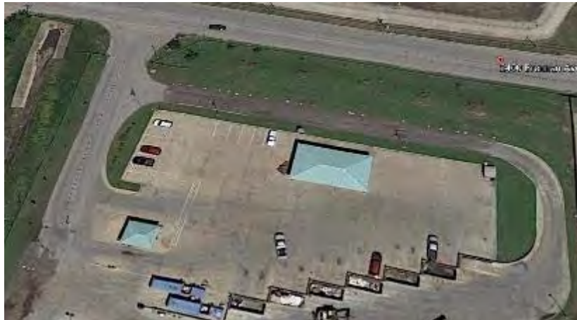
Figure 4-9 Brennan Drop-off Station
