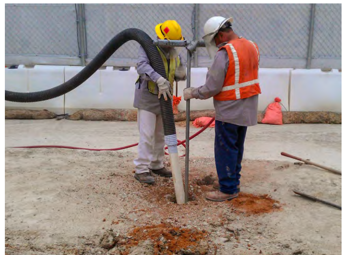
Figure 2-21. Drilling operations on a right-of-way in downtown Fort Worth to install a groundwater monitoring well, photo by City of Fort Worth.
