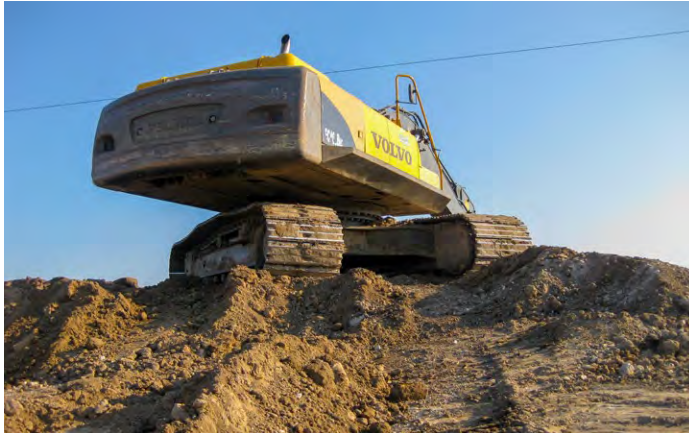
Figure 2-3. Heavy equipment is used to remove contaminated soils from sites as part of remediation activities, photo by City of Fort Worth.
