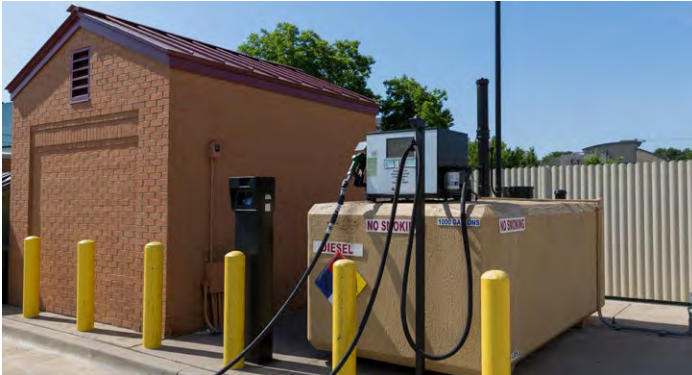
PHOTO BY CITY OF FORT WORTH
