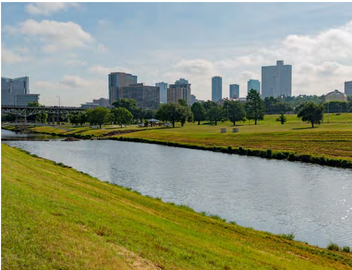
PHOTO BY CITY OF FORT WORTH
