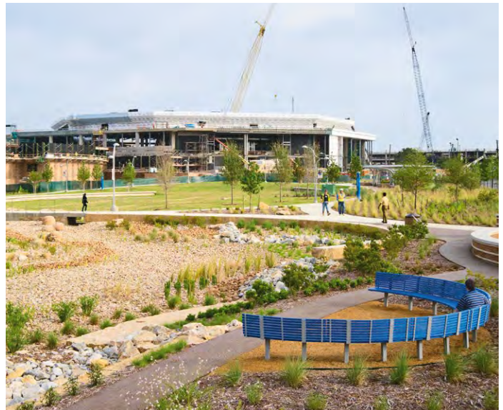
Figure 4-18. The Green at College Park on the University of Texas at Arlington campus boasts green infrastructure that captures 25 percent of stormwater and reduces sediment by 80 percent, photo from University of Texas at Arlington.
