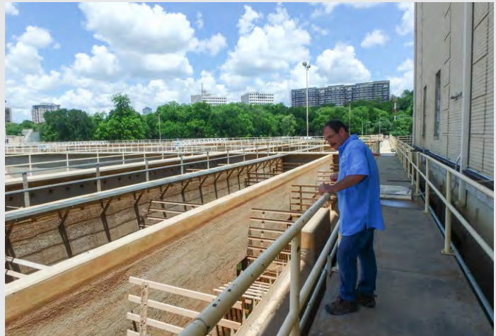
Figure 5-1. Environmental staff perform a facility audit to ensure compliance with hazardous material rules and other environmental regulations, photo by City of Fort Worth.
