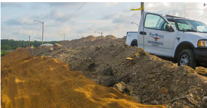
PHOTO BY CITY OF FORT WORTH
