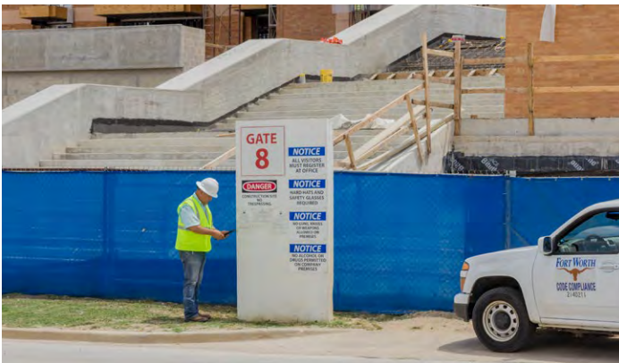
PHOTO BY CITY OF FORT WORTH
