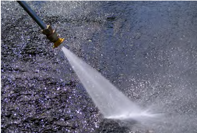
Figure 4-15. A power washer cleaning pavement.
