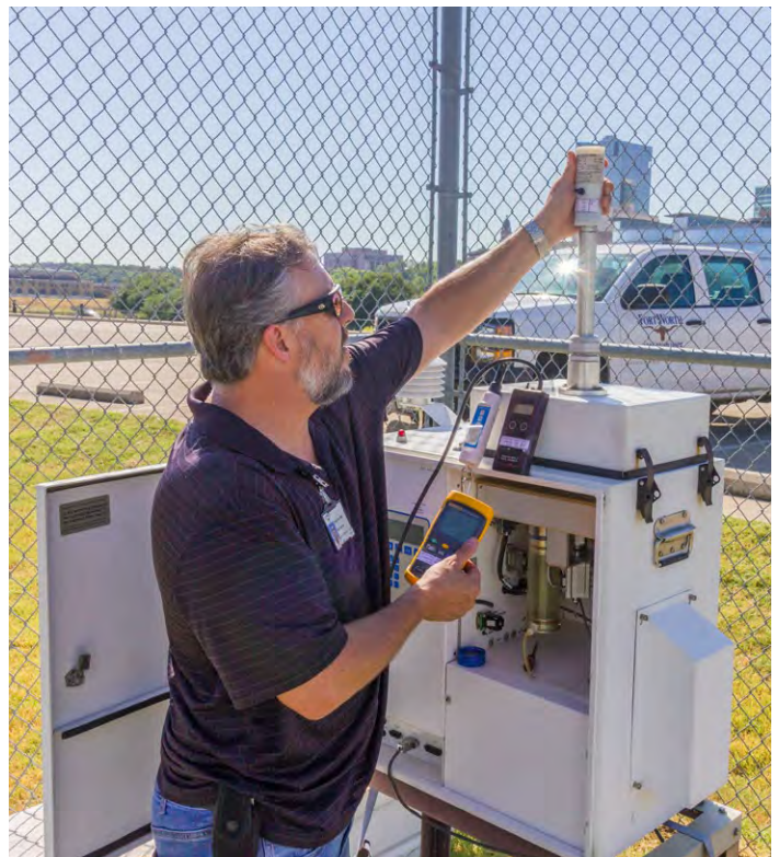
PHOTO BY CITY OF FORT WORTH
