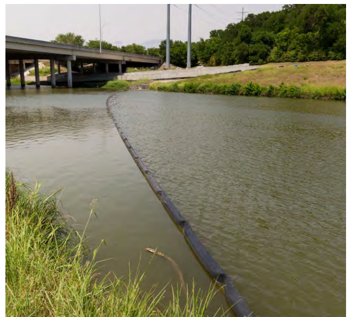
Figure 6-8. The TRWD litter boom and trash collectors across from the Clear Fork pump station, photo by City of Fort Worth.
