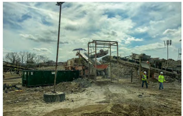
Figure 3-25. Rock crushers can cause fugitive dust if they are not operated properly, photo by City of Fort Worth.
