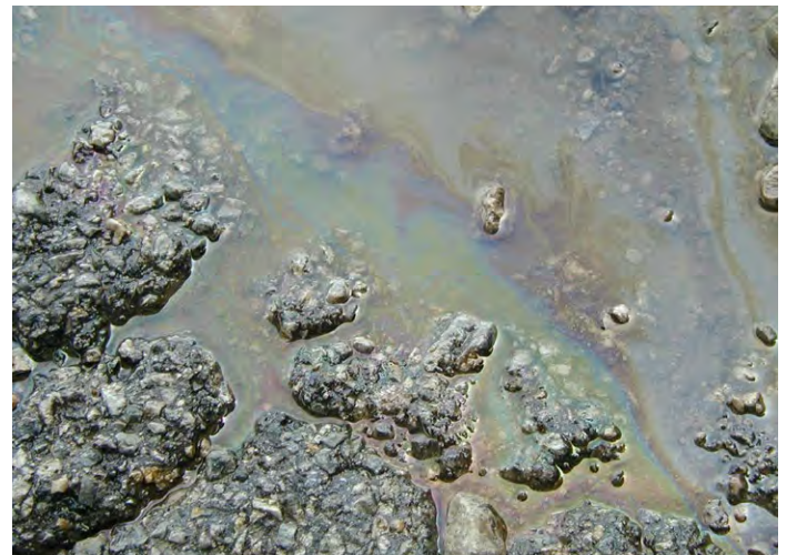
Figure 4-7. Oil sheen on asphalt.
