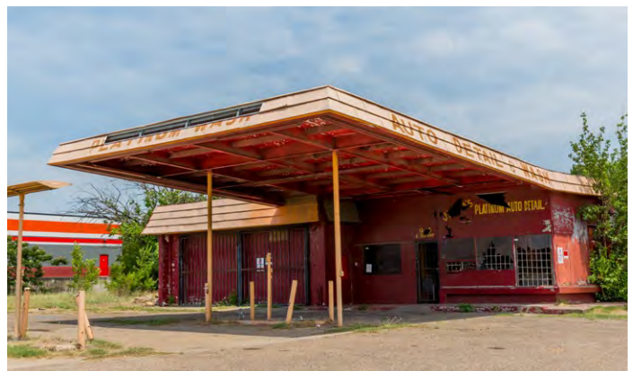
Figure 2-12. Abandoned buildings create blight and are good candidates for redevelopment, photo by City of Fort Worth.
