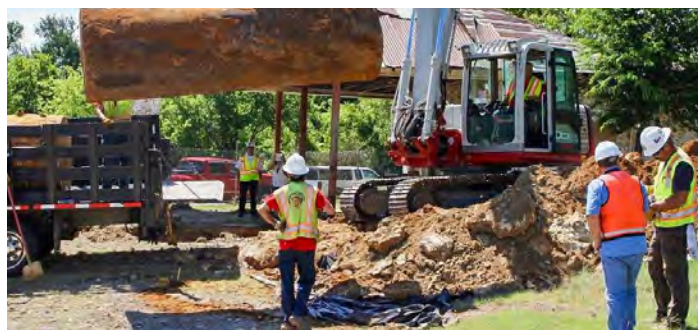
PHOTO BY CITY OF FORT WORTH
