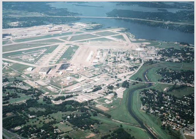
Figure 1-5. Aerial view of the Naval Air Station Fort Worth Joint Reserve Base, United States Navy, 1995. Fort Worth has a long history with the naval air program, dating back to the early 1900s when the Navy used helium from U.S. Argon to support its dirigible program.
