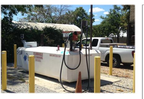
Above-ground storage tanks enhance monitoring ability and reduce the chance of undiscovered leaks and soil contamination.
