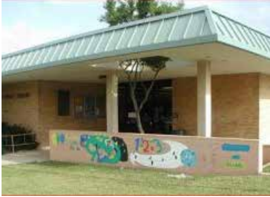
East Berry Library Council District 5 ~7,500 square feet; opened 1967
