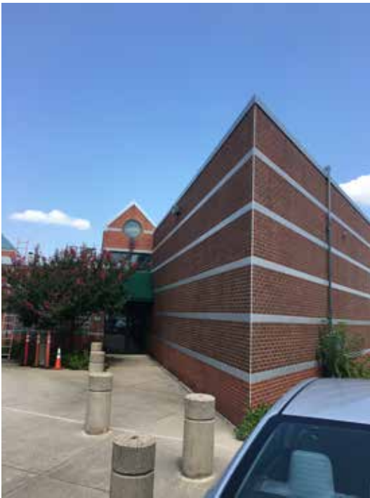
Southwest Regional Library (1987) will also require major life cycle maintenance work by 2030.
