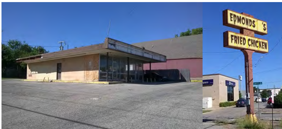
The vacant former Edmondson's restaurant is recommended for redevelopment as a mixed-use development that adheres to the Camp Bowie Form-Based Code (CB) zoning.
