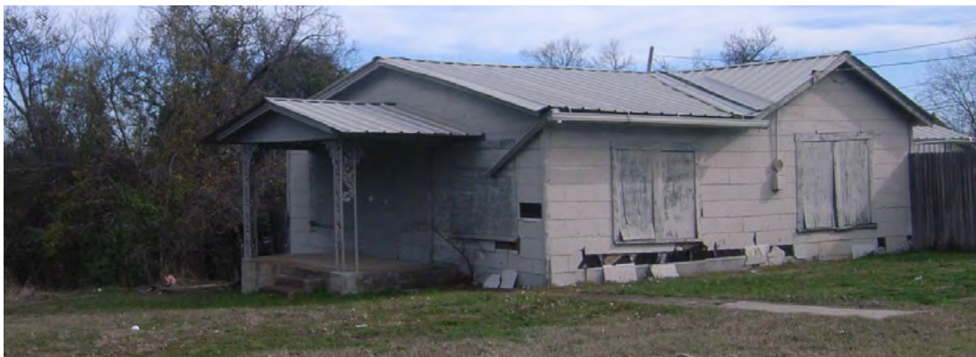
Dilapidated house in Como.
