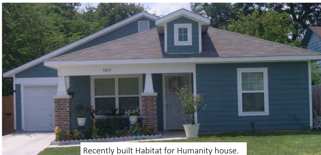
Brick façade houses.
