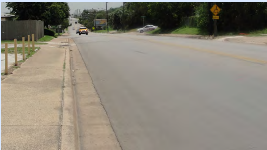
Horne Street has no traffic calming features or enhanced pedestrian crossing elements.
