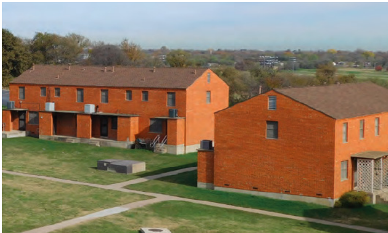
Butler Place Apartments - Public Housing
