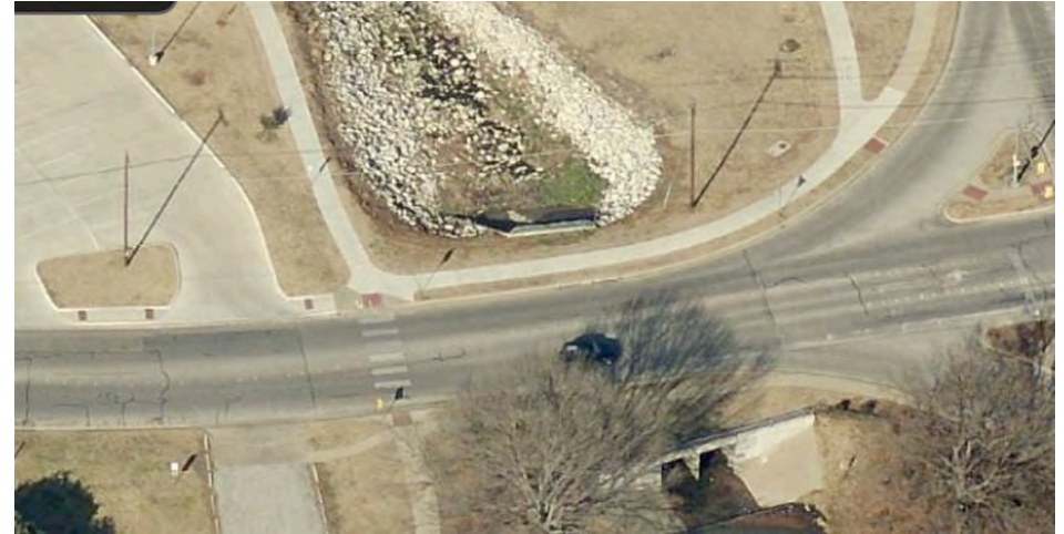
Near Intersection of South Dr. & Trail Lake Dr. * update signage/ maintain crossing markings
