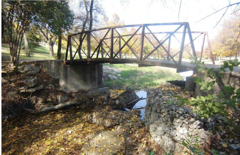
Existing Picture of Bridge at Pond
