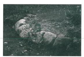
4. A single row of medium sized rocks (less than 1 foot high) might be effective at the waters edge in an area that receives a lot of use and foot traffic, such as where you access the lake or a dock.\* It is important particularly where the groundcover is grass, as grass is shallow-rooted and easily undercut by wave erosion. Install filter fabric behind the rocks so that fine soils do not wash out from behind the rocks.
