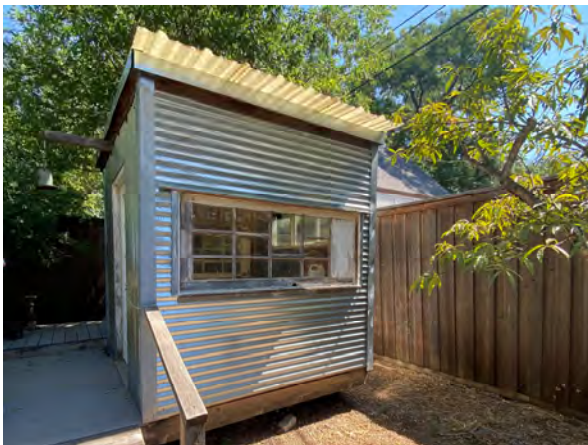
Exterior – unfinished shed
