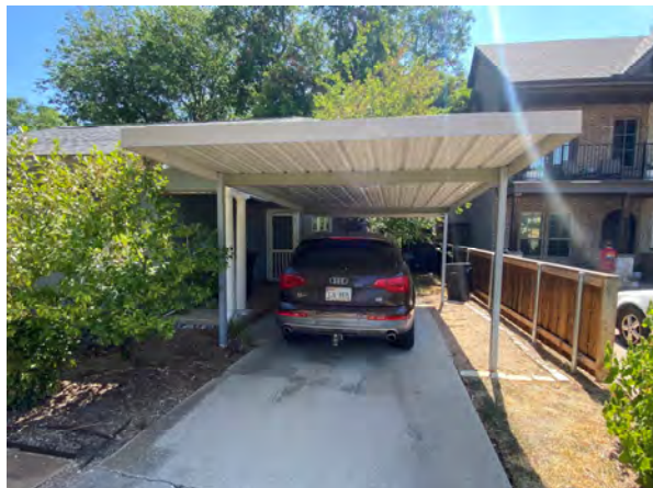
Exterior – attached carport
