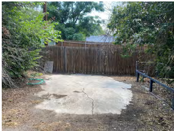
Exterior – uncovered parking area
