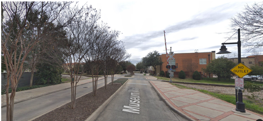
Example of an enhanced crossing in a quiet zone on Museum Way. In order to prevent drivers from deliberately driving around lowered railroad gates in this quiet zone, a median barrier is placed in the center of the roadway.
