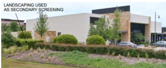
Example of compliant screen walls from the I-35 Design Overlay District’s standards and guidelines.
