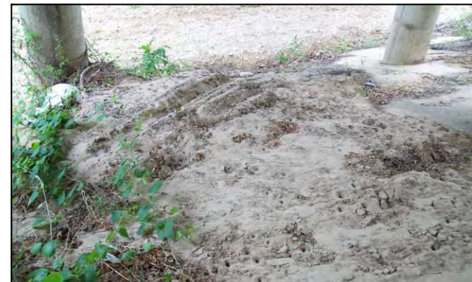
Sediment deposited on abutments from runoff at FM 1886 and Silver Creek Road
