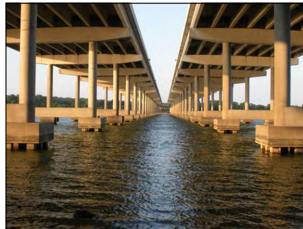
View of Lake Worth under Loop 820
