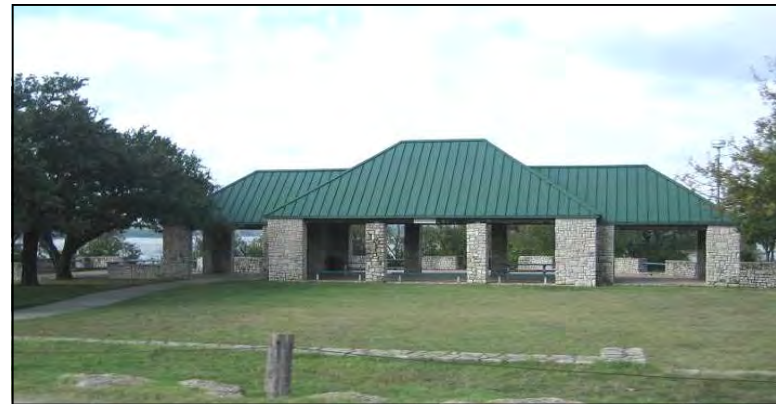
Mosque Point Park at Lake Worth
