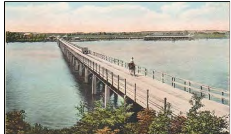
Nine Mile Bridge, Lake Worth from the Jack White Collection of Historic Fort Worth Photos, University of Texas at Arlington
