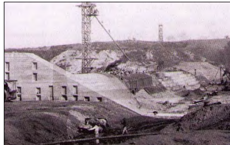
Dam construction, 1912. Freese and Nichols.
