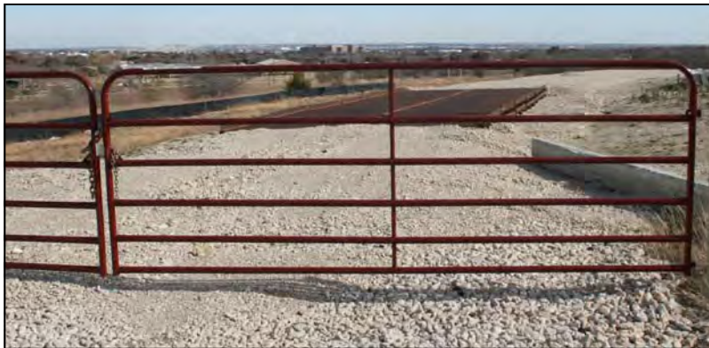
Gas well pad site
