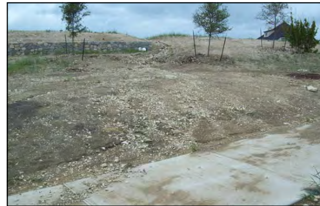
Sediment runoff from new development on White Settlement Road
