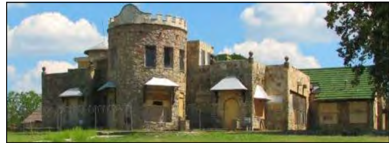
Lake Worth Castle, on the south side of the lake, could house the Hip Pocket Theatre and other cultural uses, or be redeveloped as a Bed and Breakfast
