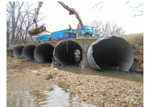
Clearing debris from storm drains.
