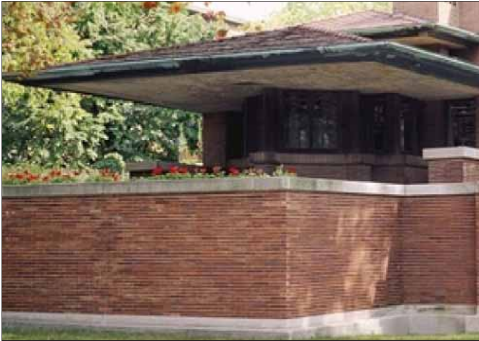
Strongly Projecting Eaves
