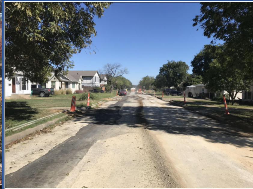
When completed, temporary pavement repair is put in place
