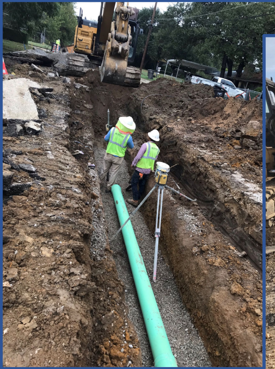
Utilities are installed first, along with new service connections to each lot
