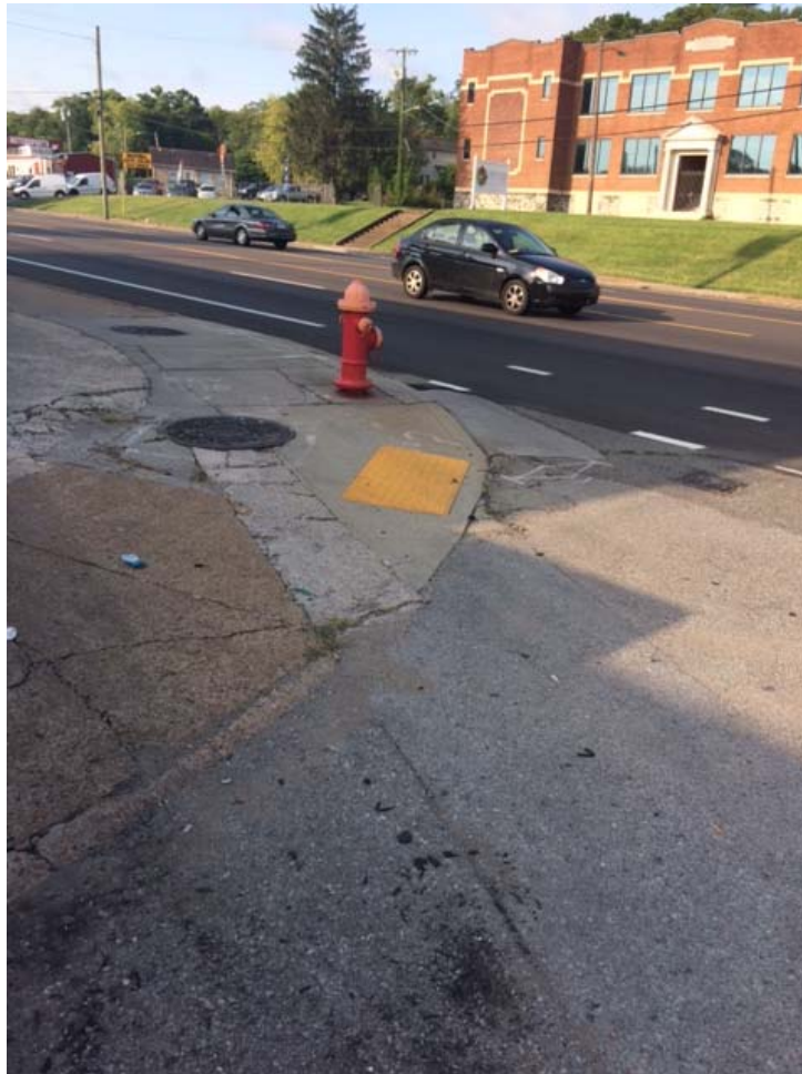
Non-Flush Curb Ramp Transition
