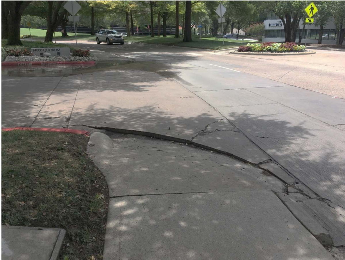
Non-Flush Curb Ramp Transition
