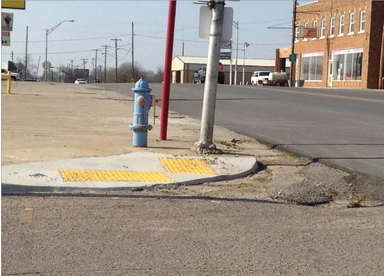
Non-Flush Curb Ramp Transition
