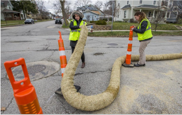
Straw Wattles used for Chicanes ; South Bend, IN; Photos: Smart Growth America
