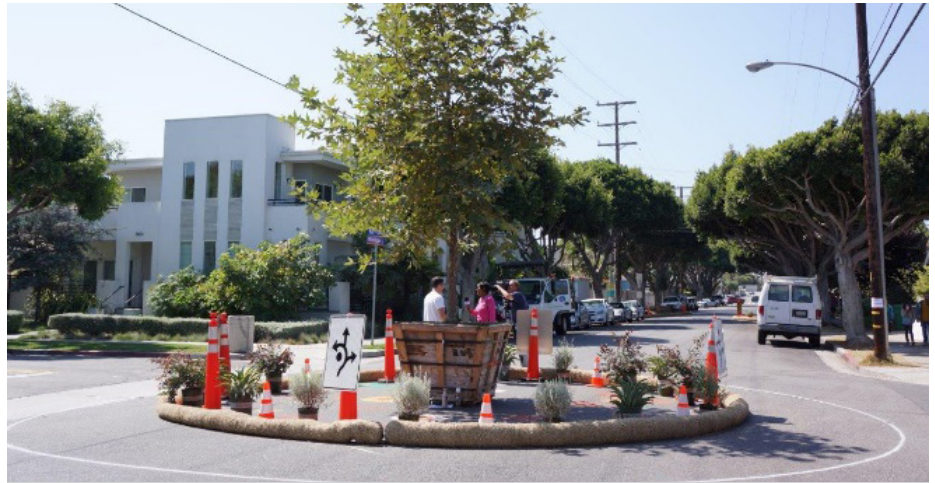
Traffic Circle made from Straw Wattle; Santa Monica, CA; Photo: Street Plans
