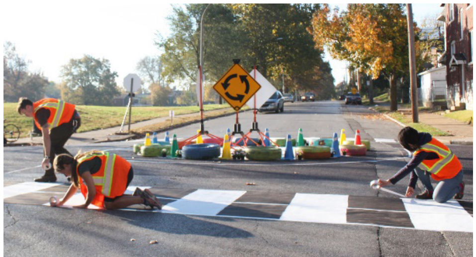
Traffic Circle made from Tires and Cones; St. Louis, MO; Photo: Trailnet
