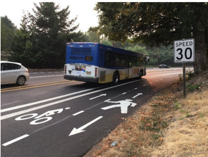
Painted Alternative Sidewalk , Portland, OR; Photo: Nick Falbo
