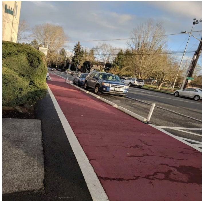
Sidewalk Extension ; Seattle, WA; Photo: Dongho Chang
