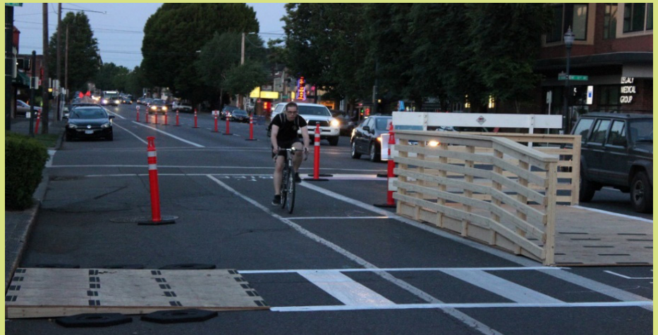
¼-inch rope was covered with 4-inch white duct tape to provide a raised edge that would be detectable with a cane.
