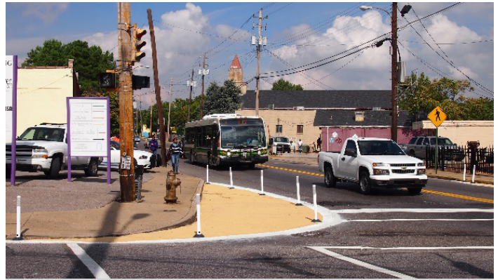
Corner Curb Extension ; MemFIX Plaza; Memphis, TN; Photo: MemFIX
