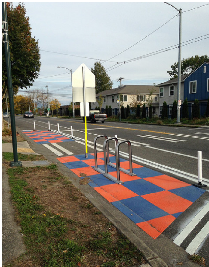
Mid-block Curb Extension ; Seattle, WA; Photo: Seattle DOT
