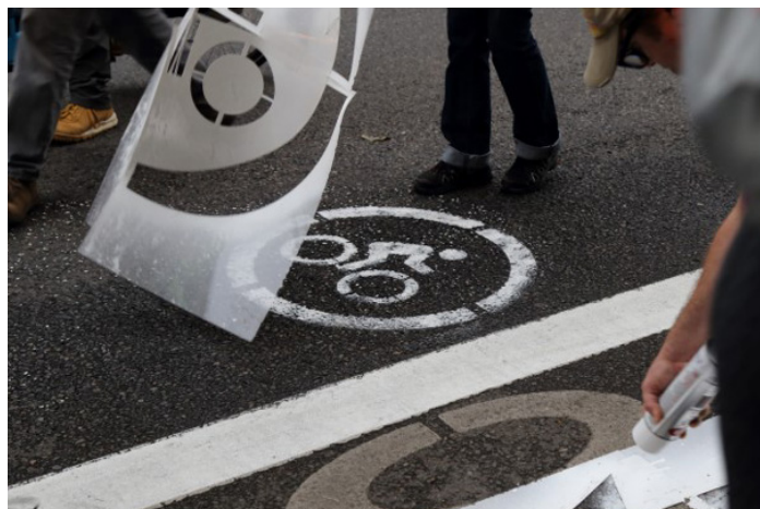
Temporary Pavement Markings in Portland, OR; Photo: Greg Raisman
