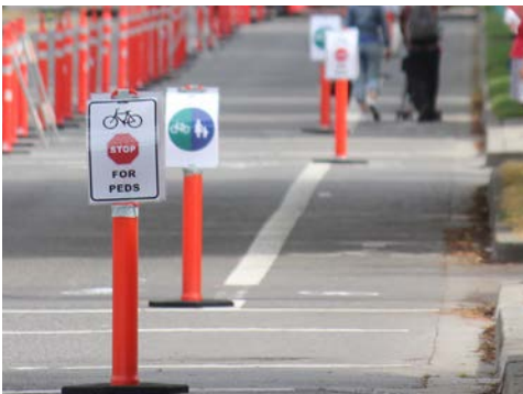
You can make homemade signs by printing and laminating 11"x17" signs. These can be zip-tied to traffic cones for a temporary sign post. ; Photo: Greg Raisman
