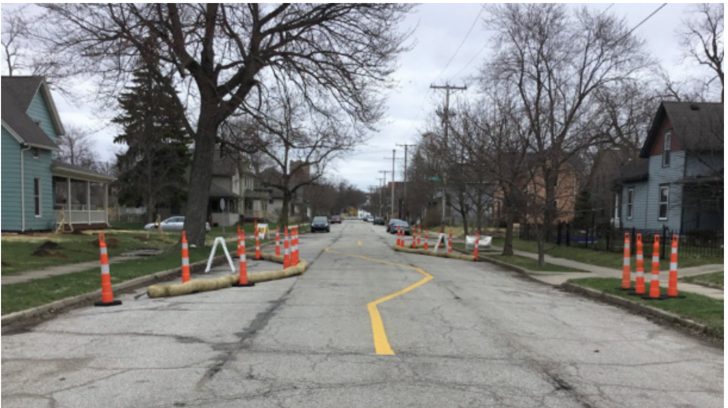
Straw Wattles used for Chicanes ; South Bend, IN; Photos: Smart Growth America
