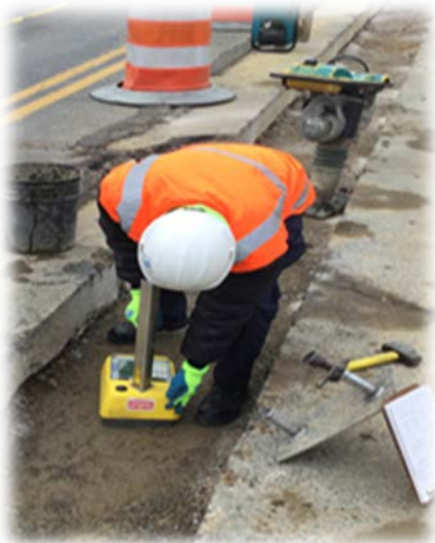
In-place density & moisture content – compacted Soil
