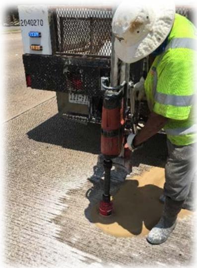
Pavement Coring
