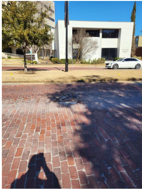
1. Identify Failed Area
