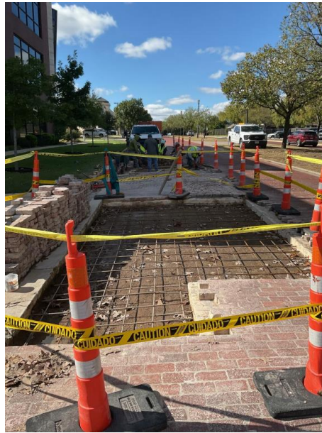
3. Install Rebar
