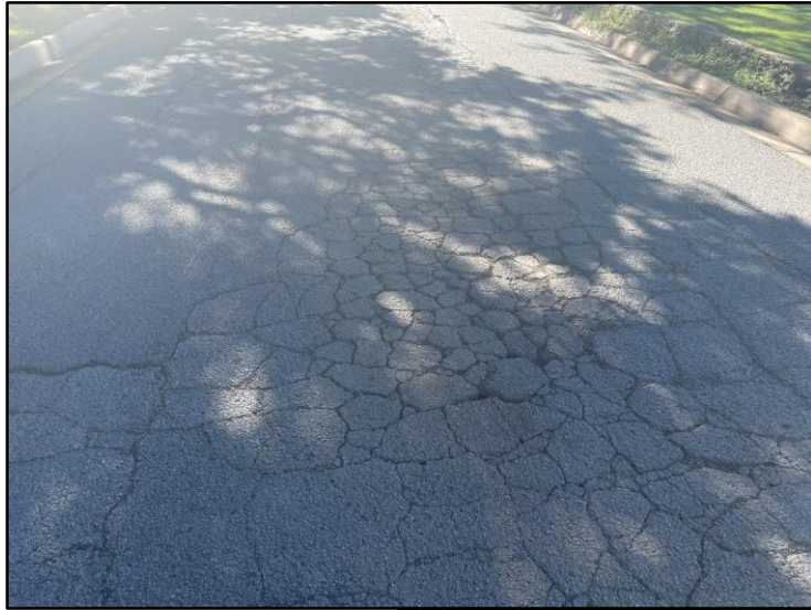
Degraded Asphalt Pavement
