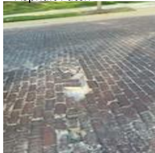
Cleaning/ Preparing for Asphalt Patch
