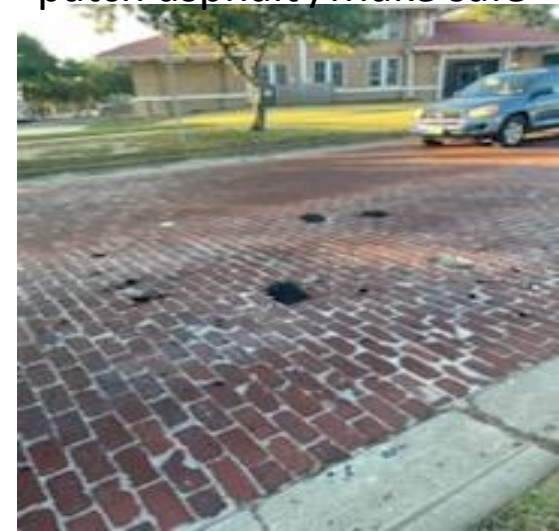
Place temporary cold patch asphalt /Make safe
