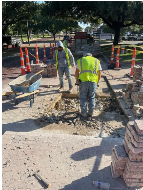
2. Remove brick and concrete
