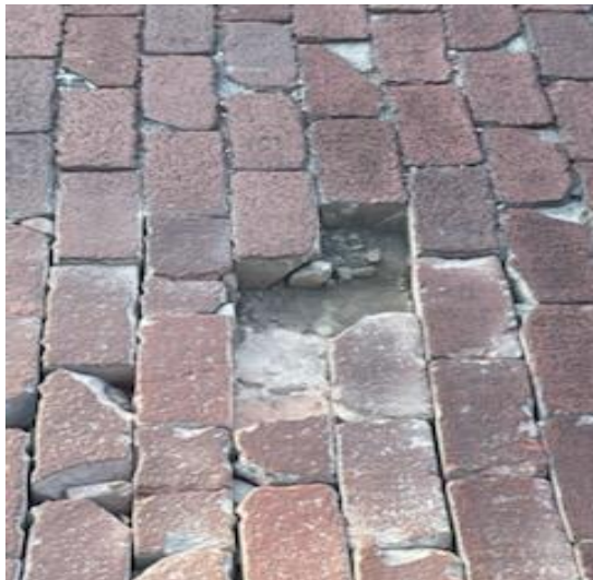
Removal of Lost/Lose Bricks
