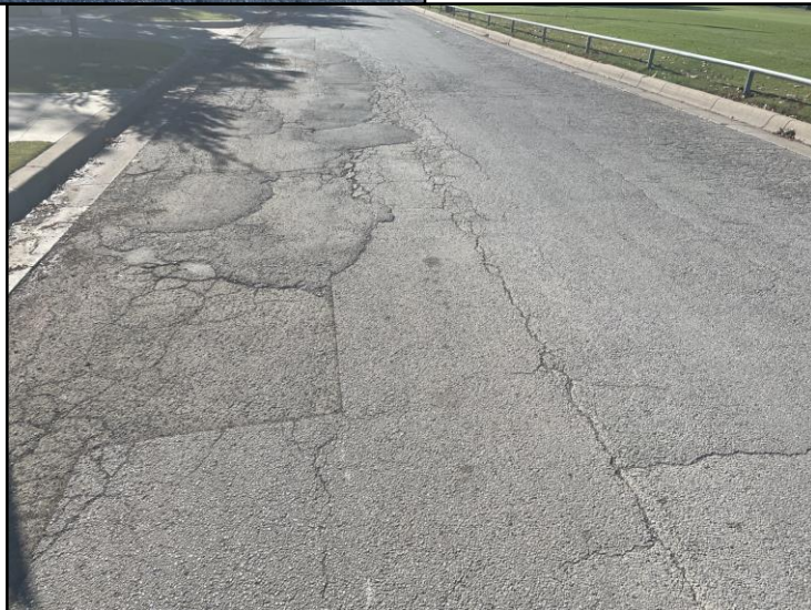
Degraded Asphalt Pavement
