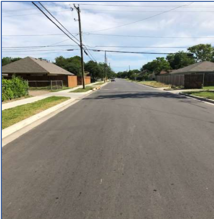
New Pavement and Concrete Curb & Gutter
