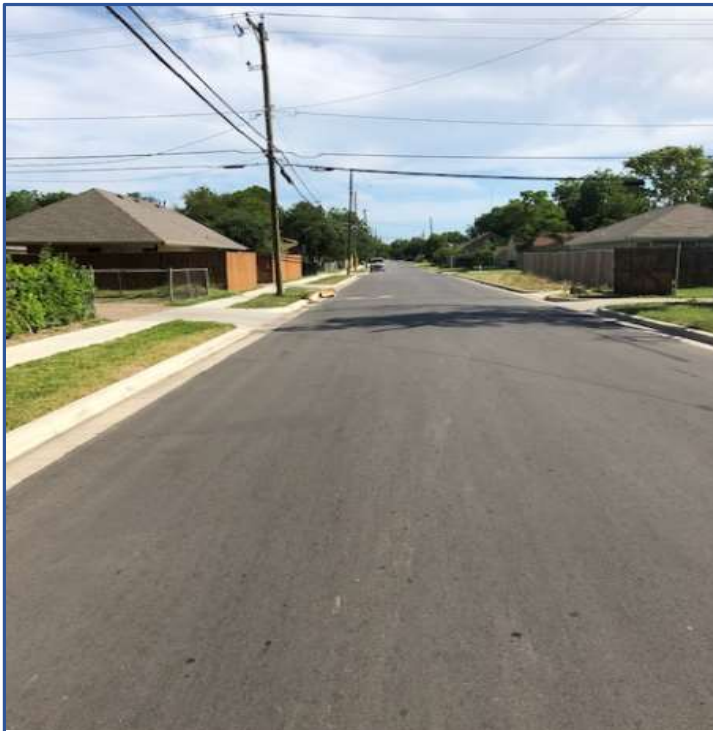
New Pavement and Concrete Curb & Gutter
