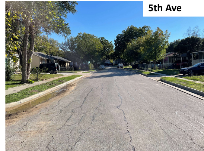
Damaged Asphalt Paving
