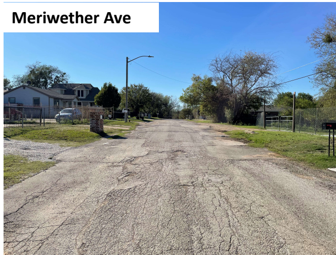
Damaged Asphalt Paving
