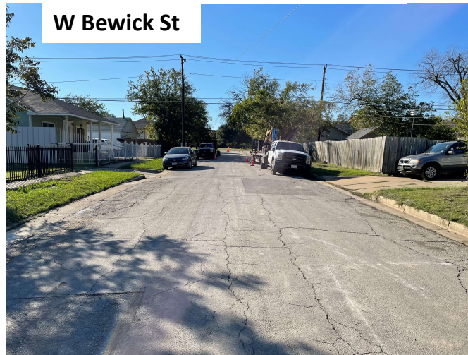
Damaged Asphalt Paving
