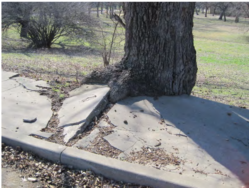
TREE ROOTS CRUMBLING A SIDEWALK
