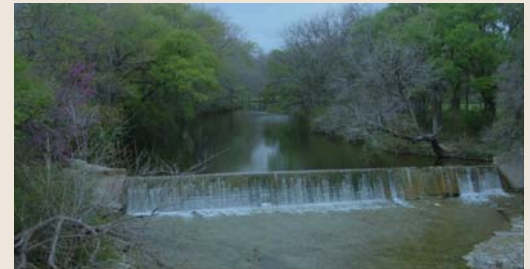
One of several low water dams along Mary's Creek
